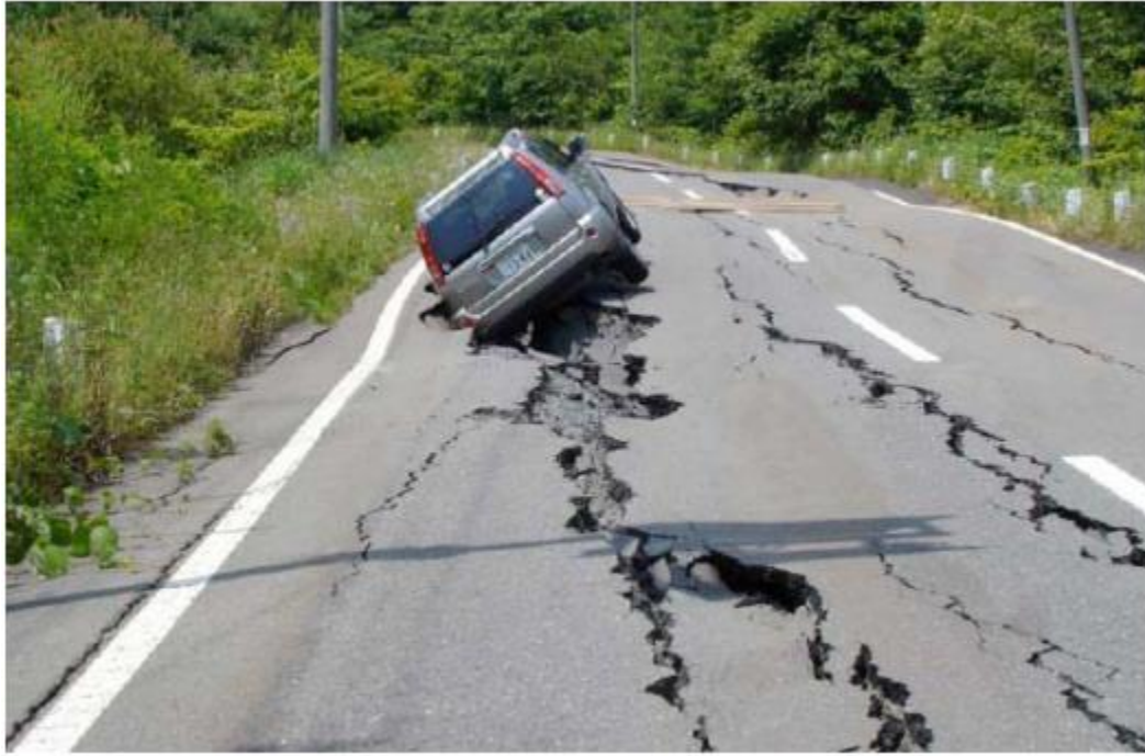
Figure 3.5 Road Embankment Damage Caused by Lateral Slumping During the 2008 Iwate Miyagi-Nairiku Earthquake, Japan (Adopted from SYNER-G Project 244061, 2011)
