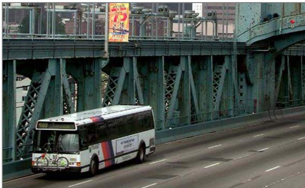
Figure 2.5 Bridge as Barrier for Cycling (bikewalk.org, 2004)
