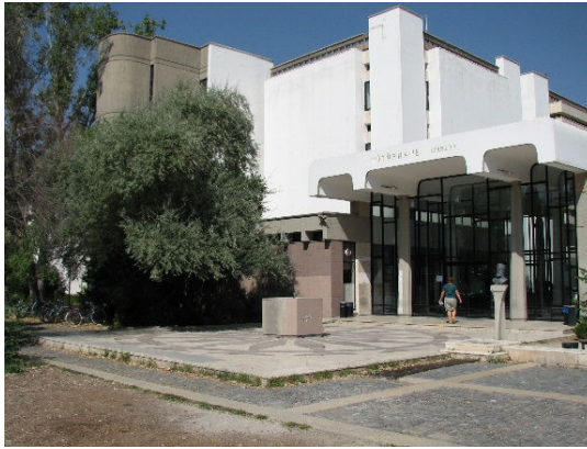
Figure 18: Variations in the surface finish in front of the Library Building
