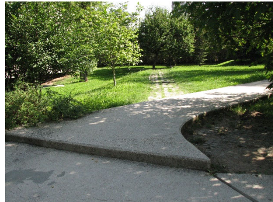
Figure 8: The continuity in circulation is severed by minor level differences
