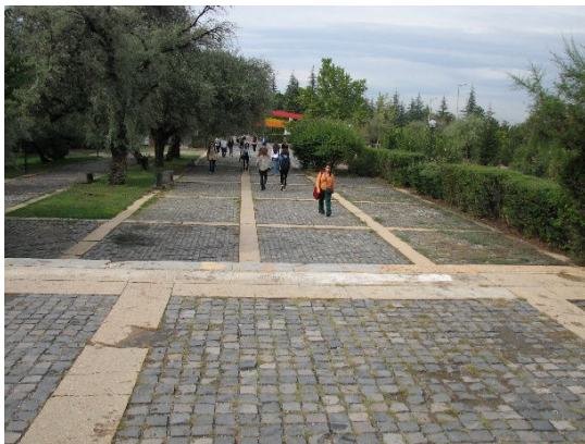
Figure 16: Paved surface finishing of the Pedestrian Alley, as the main public realm on campus
