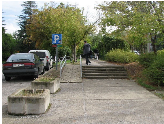
Figure 14: A steep ramp not linked with an accessible route results in its disuse
