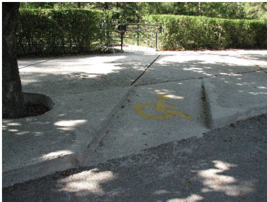
Figure 5: A curb ramp with an appropriate sloped and surface quality
