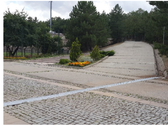
Figure 34: Sloping surface with changing tactility
