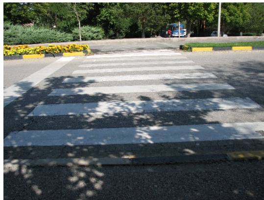
Figure 23: The participants cannot use, or even know about the displayed crossing, located at the centre of most commonly used area, due to a lack of perceptible information indicating its presence.
