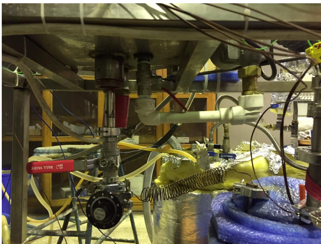
Figure 4.23 Photograph of throttling valve and the capillary tube installed between condenser and evaporator.
