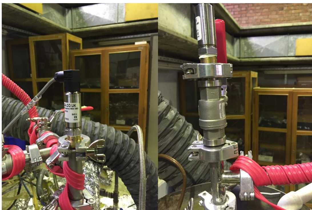
Figure 4.29 Photograph of the pressure transducer installed to the condenser
