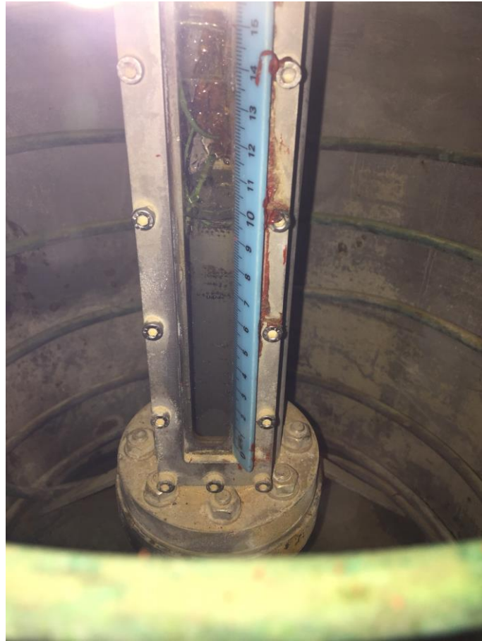
Figure 4.20 The sight glass of the condenser canister
