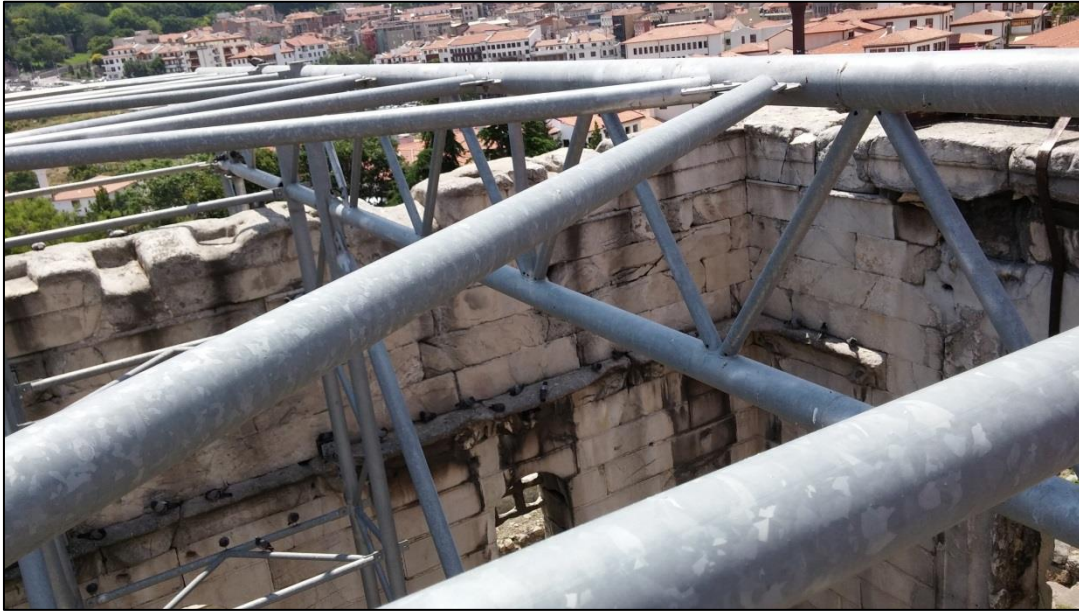
Figure A.9: Temple from atop the northern isolated wall, looking at the intersection of the southeastern wall and the gate section. The slots where most probably the ancient wooden beams were placed are visible.
