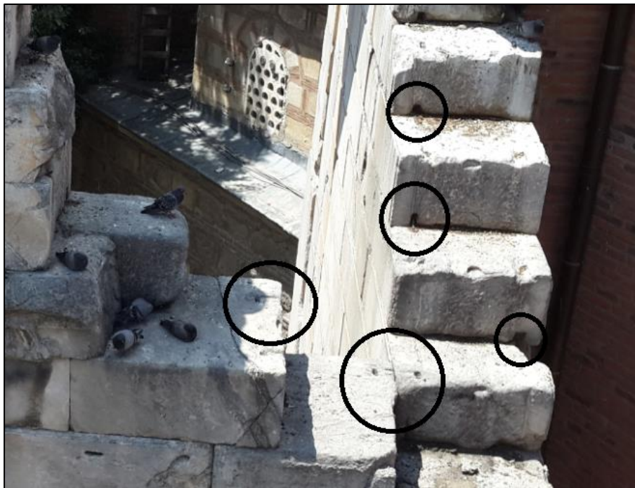
Figure 1.9: Marks showing the application of Opus Revinctum on the temple
