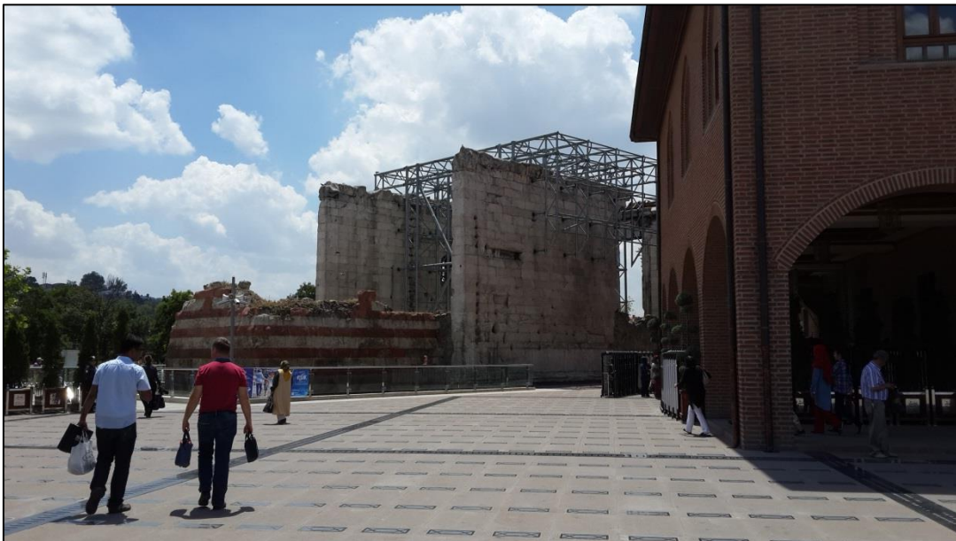
Figure A.3: General view from the northern vantage point, the northern isolated wall in the front
