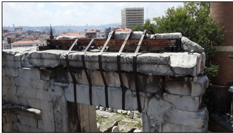
Figure 1.12: Door lintel in a deteriorated state. Intervener and the date of intervention are unknown.
