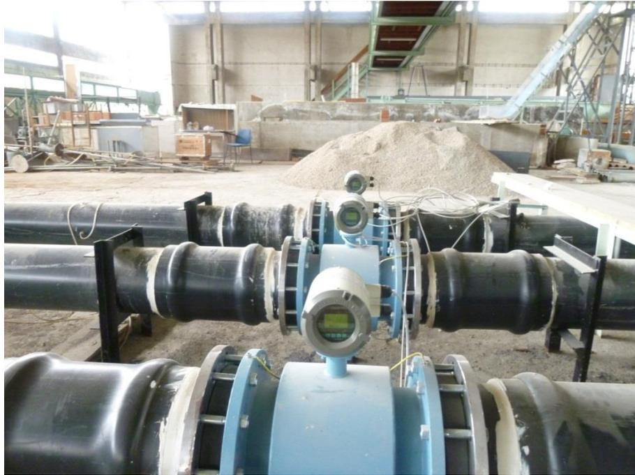
Figure 4.7 View of the electromagnetic flowmeters mounted on the water intake pipes
