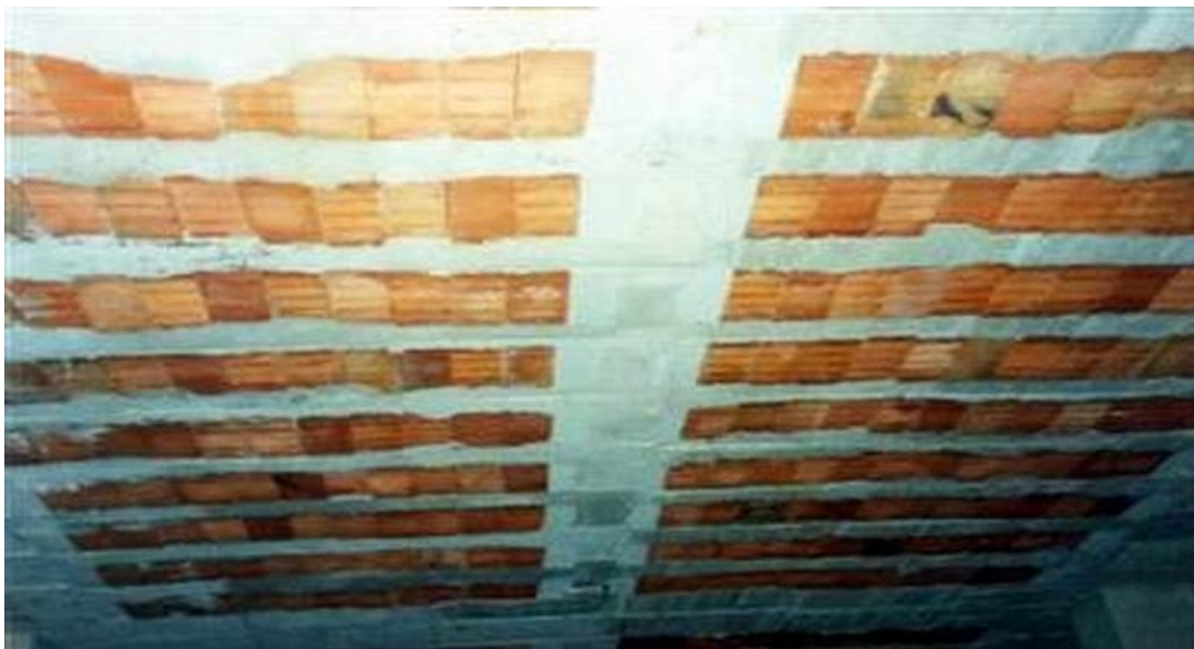
Figure 1.1. Wide-beam infill joist block one-way slab (asmolen)
