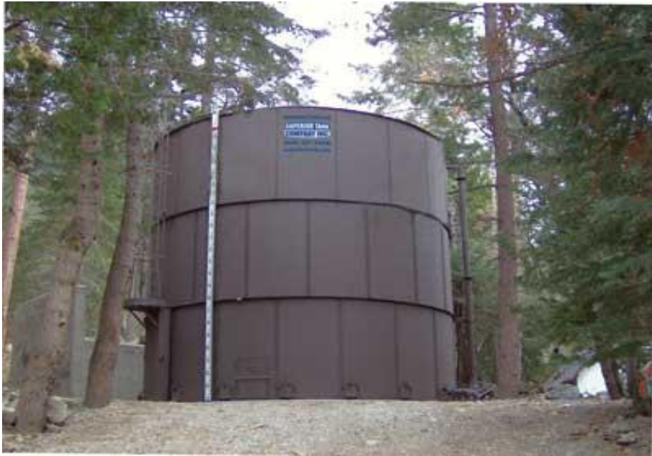
Figure 3 A Storage Tank with Cylindrical Shape (“Water storage tanks - WaterWorld,” 2015, November 20)
