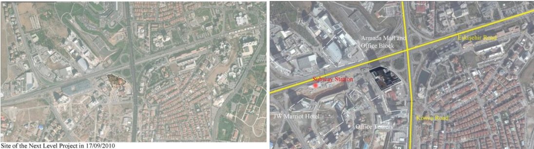
Figure5.4: Site of the Next Level Ankara Project, old and new views
