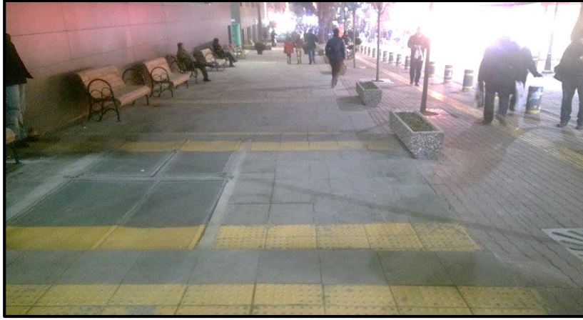
Figure 3. 26 Ground Pavements for Visually Handicapped People (Source: Author' Archive, 2015)
