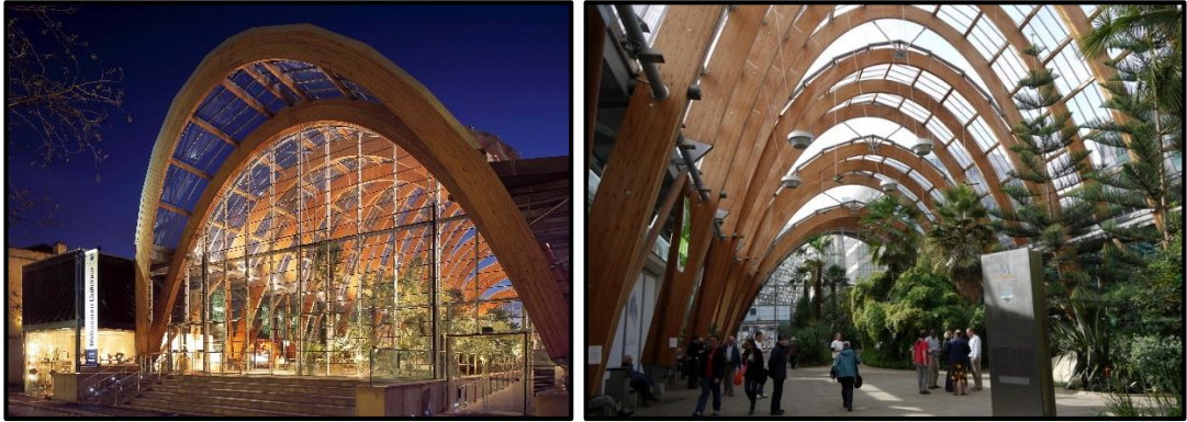
Figure 2. 9 Winter Garden in Sheffield (Source: openbuildings.com, 22.06.2015)
