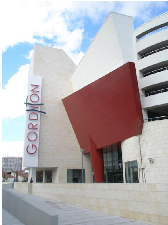
Figure 3 : Gordion Shopping Mall (Chapman Taylor Architects, 2015, retrieved on July 20 th , 2015)
