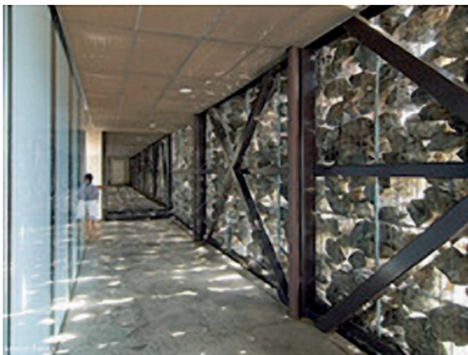
Figure 6: Walls of Dominus Winery ( http://dominusestate.com/wp-content/uploads/2015/03/architecture.jpg/ , Retrieved July 9, 2015)
