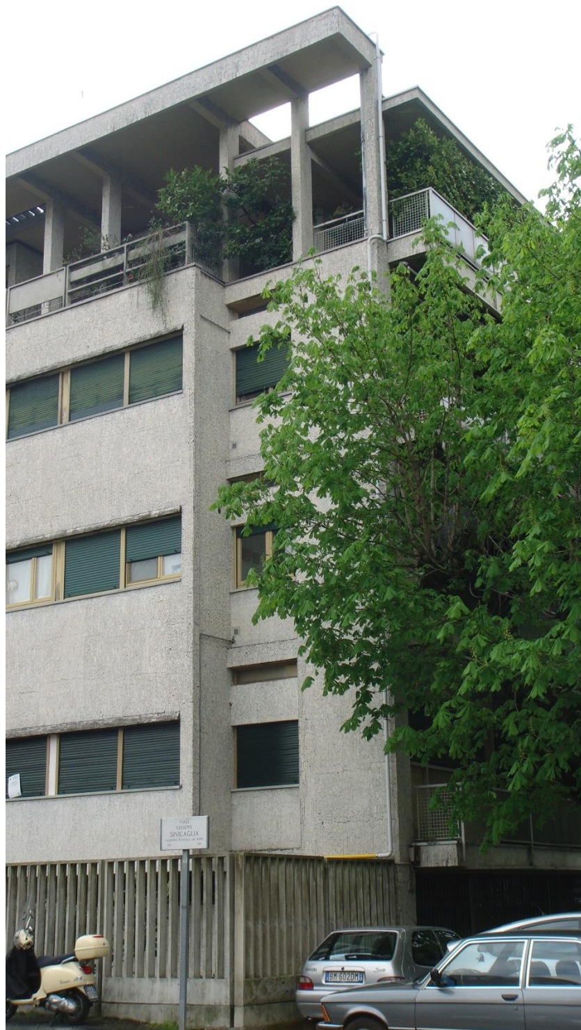
Figure 39. Casa Giuliani-Frigerio, Disjunctions at the Roof Level. Photo by the author.
