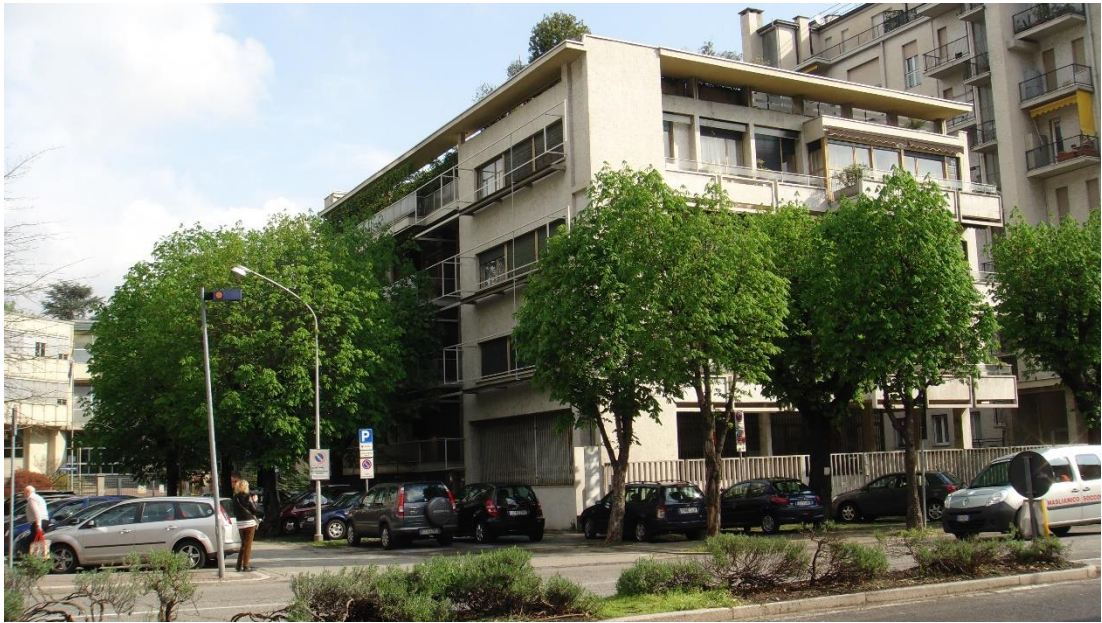
Figure 36. Casa Giuliani-Frigerio, Como, Italy. Photo by the author.
