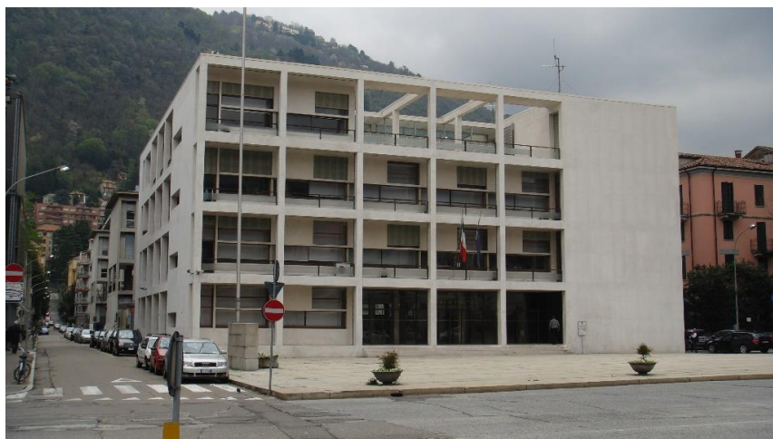
Figure 10. Casa del Fascio, Como, Italy. Photo by the author
