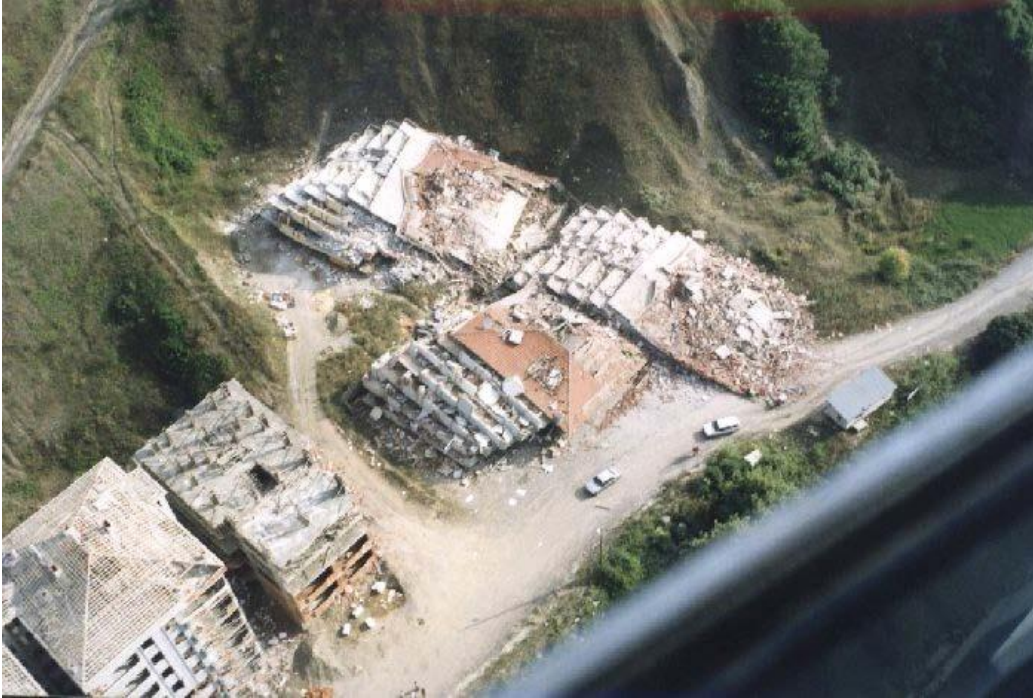
Figure 1.1 Aerial views of a few typical RC-MRF buildings in Gölcük. Traditional and faulty construction practices with limited interstory drift capacity under near-fault ground motion led to structural instability and excessive damage, including full collapse. [Courtesy of http://www.koeri.boun.edu.tr/depremmuh/eski/eqspecials/kocaeli/golcuk.htm ]
