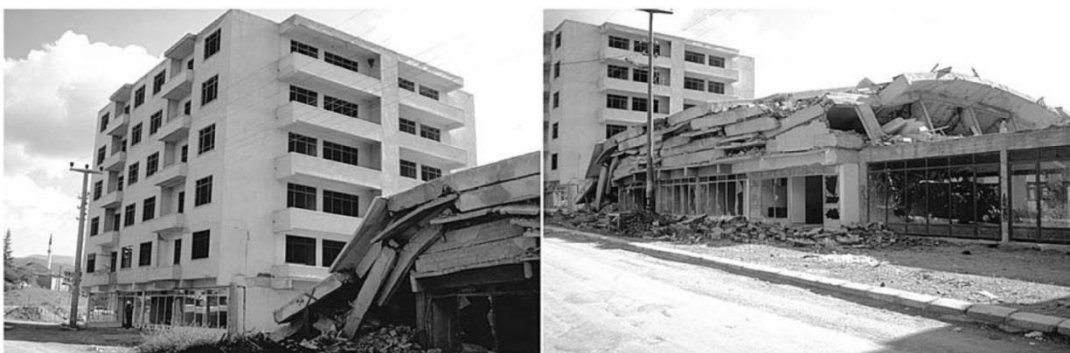
Figure 1.2 Changeability of two adjacent, similar building responses proceed from different limit states; post-yielding hysteresis behavior pattern; and interstory drift capacities (Sezen et al., 2003)
