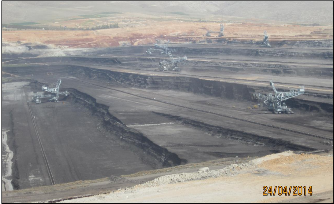
Figure 14. Lignite excavation benches in the Sector A
