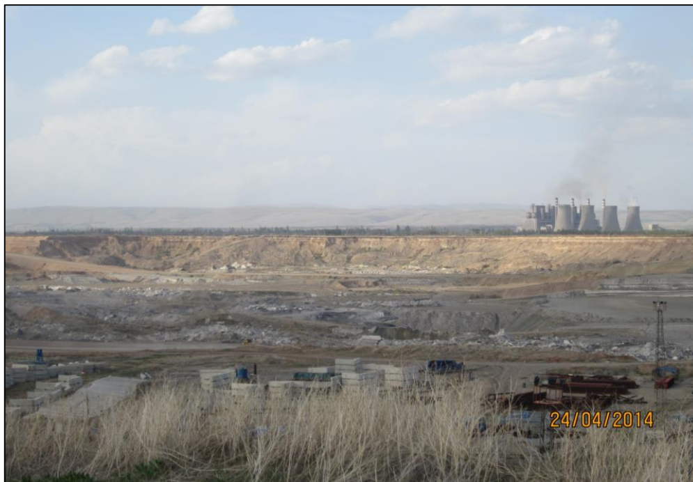
Figure 17. Slope failure at the north-west slope of the Sector B
