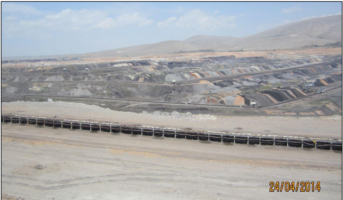
Figure 15. Waste dump site and waste spoils in the Sector A
