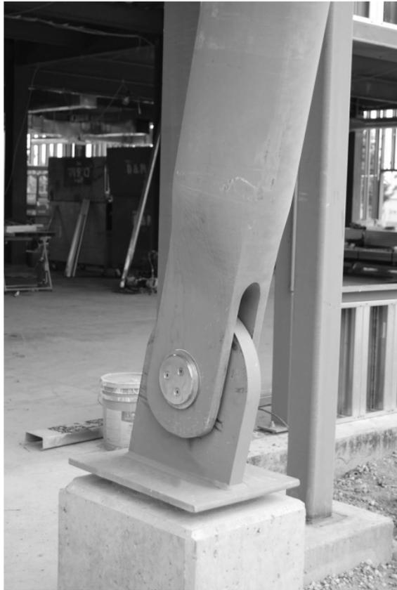
**Figure 41. Pin ended circular hollow section column [21]**
