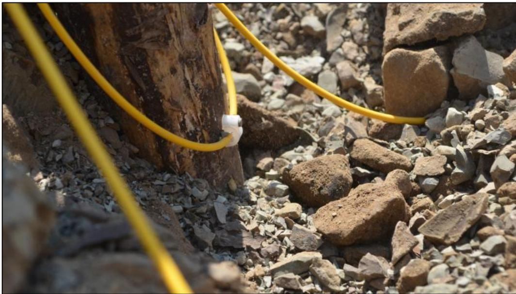
**Figure 49: Close up view showing fixing of the cable on a wooden pole**
