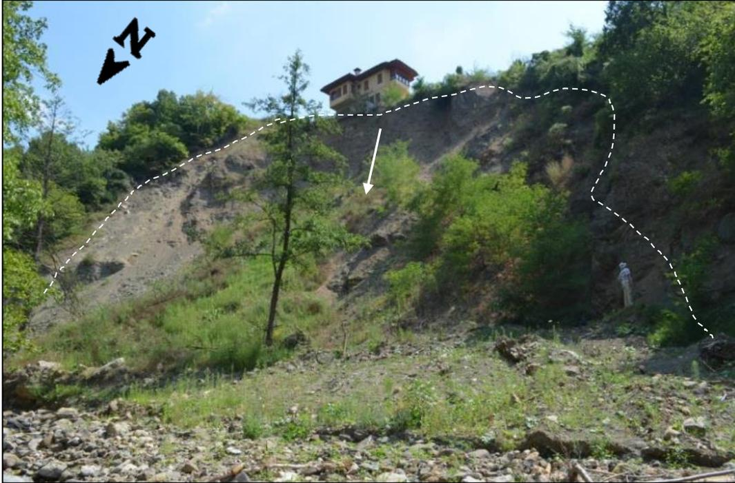
**Figure 3: General geometry of the landslide and the house affected**
