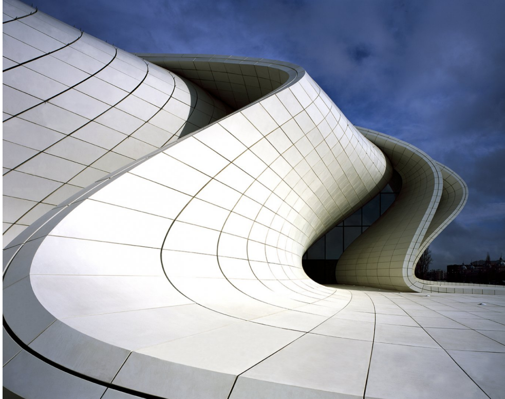
Figure 2.2 Heydar Aliyev Centre by Zaha Hadid Architects
