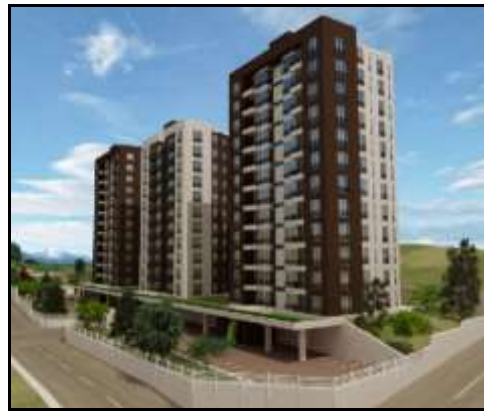
Name of Housing Estate: Pelit Yaşam Number of Housing Units: 72
