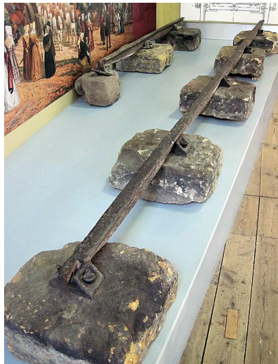
Figure 2.2: A Section of Rail Tracks on Stone Block Sleepers (Source: gerald-massey.org.uk/Railway/c10_construction_(IV).htm )
