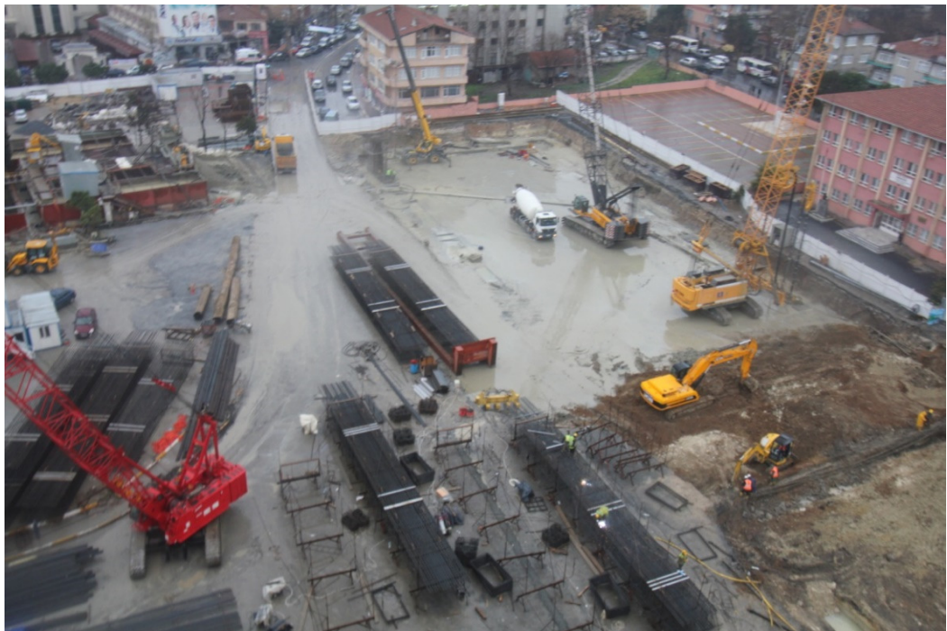
Figure 3.3. Bağcılar Station Excavation Field
