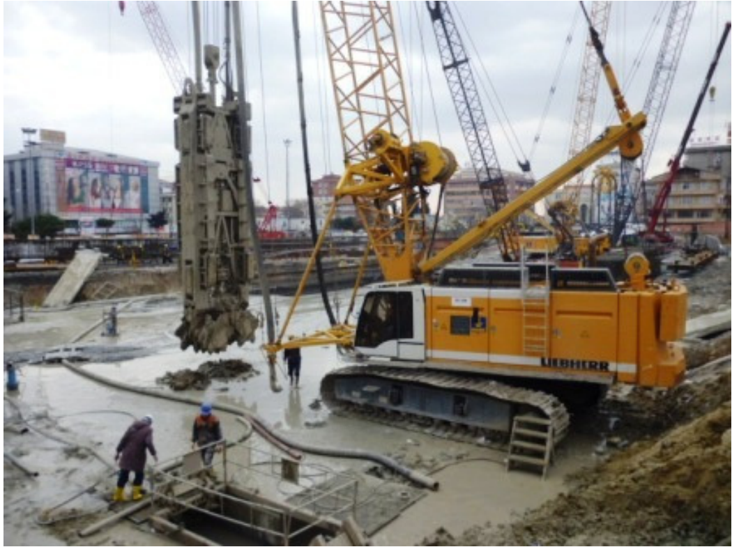
Figure 3.2. Bağcılar Station Diaphragm Wall Equipment
