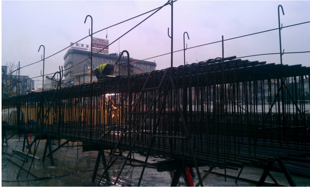
Figure 3.4. Bağcılar Station Diaphragm Wall Reinforcements
