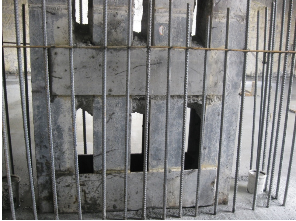
Figure 3.6. Bağcılar Station Steel-Concrete Composite Column
