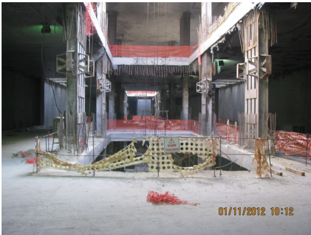
Figure 3.5. Inside View of Bağcılar Station during Construction
