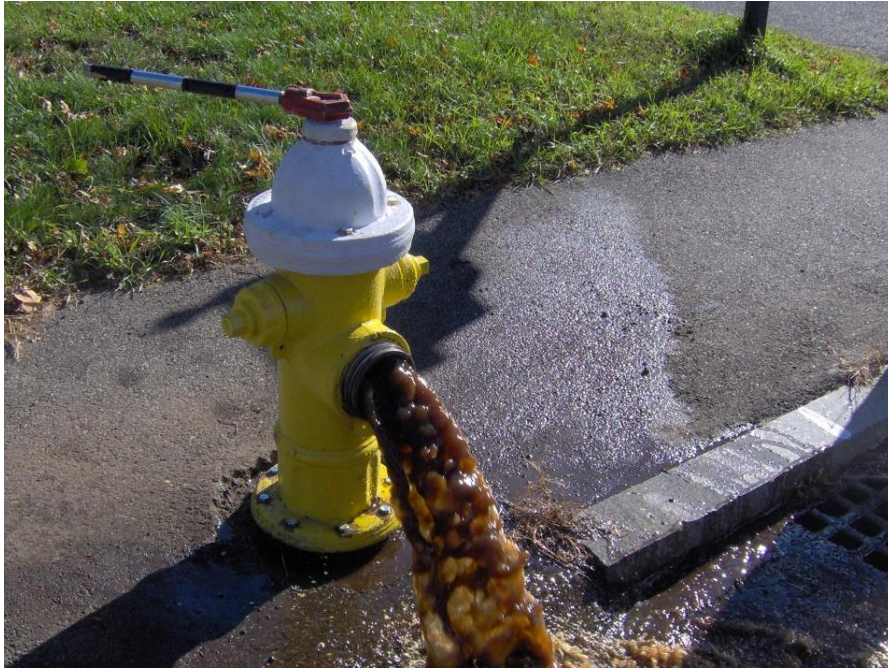
Figure 2.5. Flushing Operation (Needham Water and Sewer Division, n.d.)
