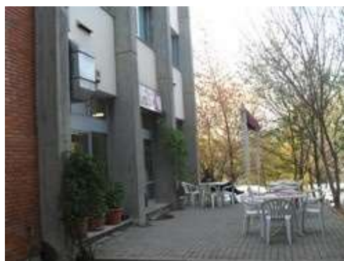
Figure 4.5.4 Photographed by GEOE11
