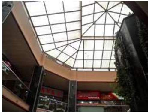
Figure 4.8.21 Photographed by GEOE2
