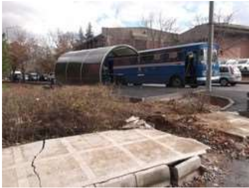
Figure 4.8.36 Photographed by GEOE9
