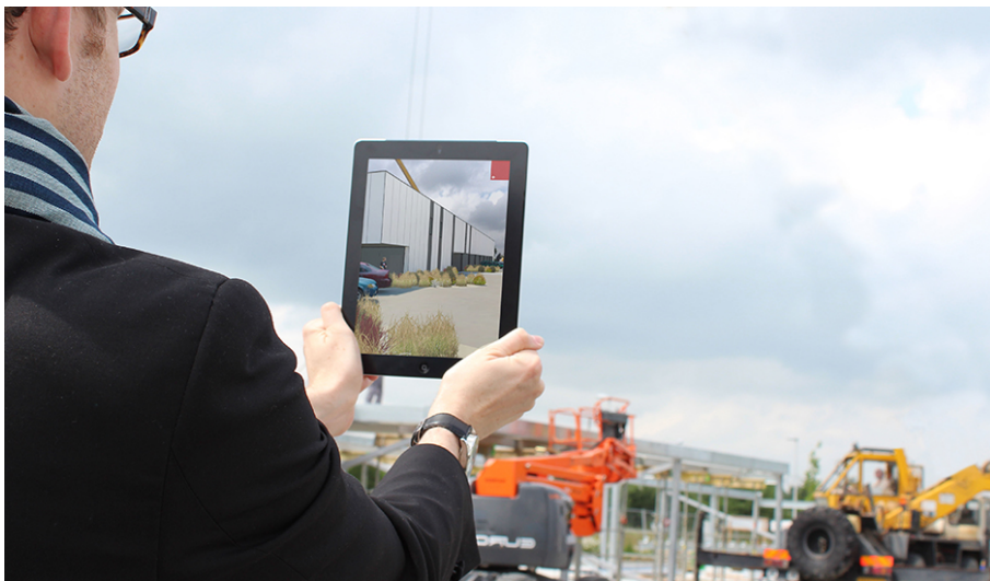
Figure 2.27: Viewing of the construction site with Urbasee [34]
