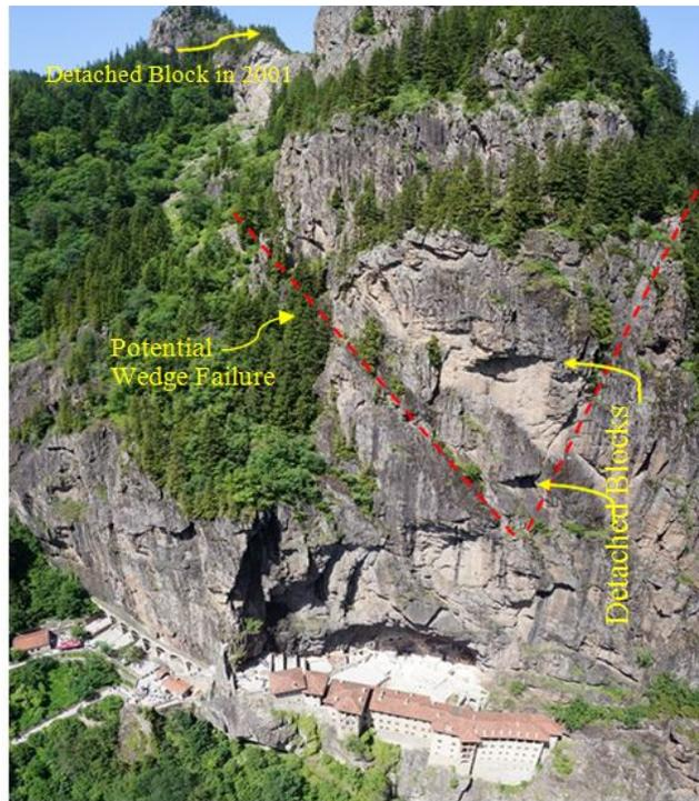
Figure 4.5 –Potential wedge failure and detached blocks from it.
