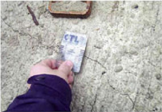
Figure 2.9 Thermal cracks in a bridge deck (adopted from <http://www.cement.org>)
