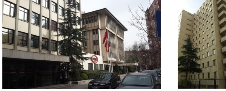
Figure 63 Tall buildings along the main road
