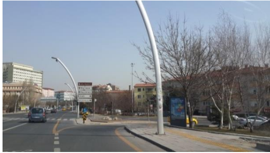
Location of the station
