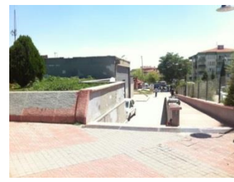
Stairs and ramps
