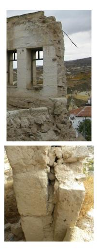
Figure 3. 34 Double sided walls constructed with cut stones
