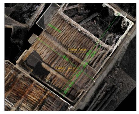
Figure 3. 61 Earth roof on timber beam superstructure (Orthophoto)
