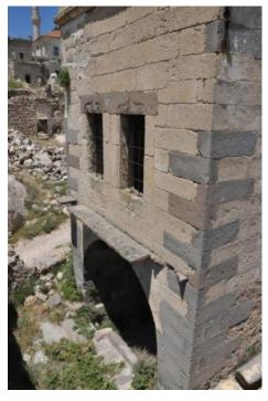
Figure 3. 8 Kepez stone on corner and lintels
