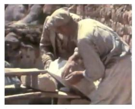
Figure 4. 13 Voussoirs are placing with formwork<sup>9</sup>
