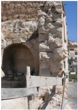
Figure 3. 36 Double sided walls constructed with rough cut stones-ground floor wall
