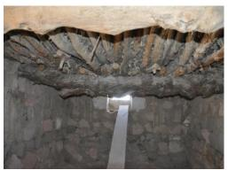
Figure 3. 55 Natural shaped beams
