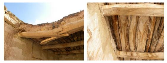
Figure 3. 65 Earth roof on flat superstructure
