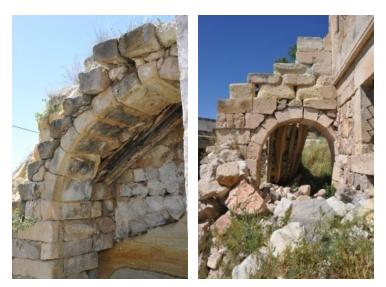
Figure 3. 80 Staircase arch supported and timber beams
