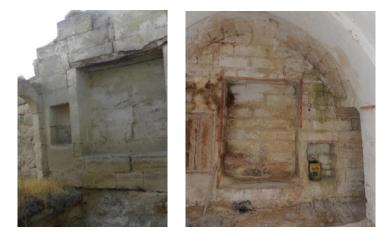
Figure 3. 149 Yüklük spanned with timber lintel
