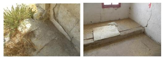
Figure 3.9 Sal stone usage on courtyard and floor covering
