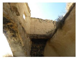
Figure 3. 77 Transition between rock and masonry by timber beams
