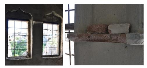
Figure 3. 153 Projected flat lambalık between two windows
