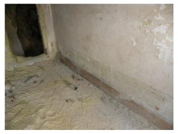
Figure 3. 132 Timber seki and timber plate traces on wall
