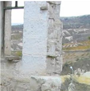
Figure 3. 35 Double sided walls constructed with cut stones
