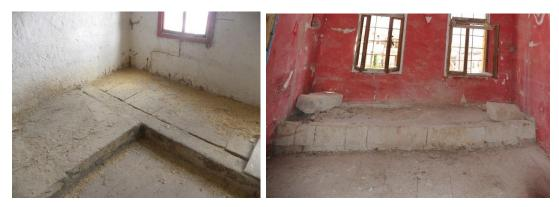
Figure 3. 129 (left) 'L' shaped stone sedir (right) Stone sedir
