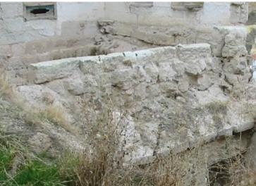
Figure 3. 37 Double sided walls infill with 'sillez' - Supporter wall of vault
