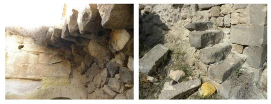
Figure 3. 84 Type-2 staircase, steps are projected
