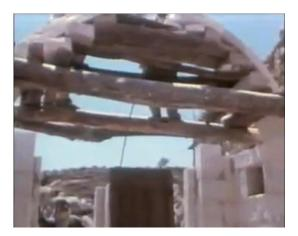
Figure 4. 12 Formwork of vault<sup>8</sup>
