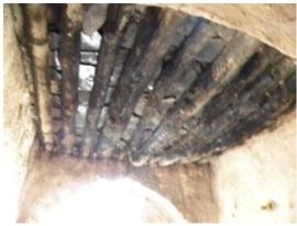
Figure 3. 57 '*Saylak*' stone above the timber beams
