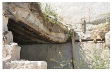
Figure 3. 10 Kevek stone usage on timber beam ceiling
