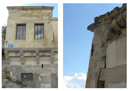
Figure 3. 12 Iron tie-bar and window railings
