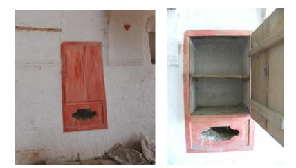
Figure 3. 147 Built-in cub-board with drawer
