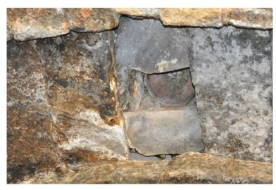
Figure 3. 69 Traditional hand-made terra cotta bowl insert to the opening
