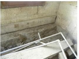
Figure 3. 127 Projected stone usage Instead of opening hollow for *sedir*
