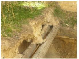
Figure 3. 56 '*Saylak*' stone above the timber and soil layer on top of them
