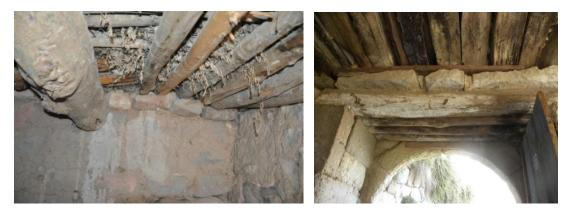
Figure 3. 11 Timber usage on ceiling and to span door opening
