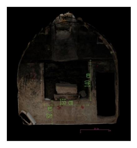
Figure 3. 151 Orthophoto elevation of yüklük
