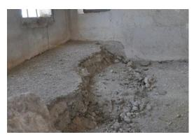
Figure 3. 128 Soil and stone pieces infill of sedir
