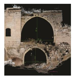
Figure 3. 46 Upper floor widest vault arch with three rows of cover arch
