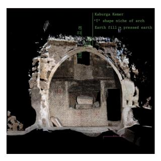
Figure 3. 59 Orthophoto of earth roof filled with 'şillez'
