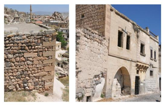
Figure 3. 30 Rough-cut stone lateral façade and cut stone corners Cut stone used in main façade of building
