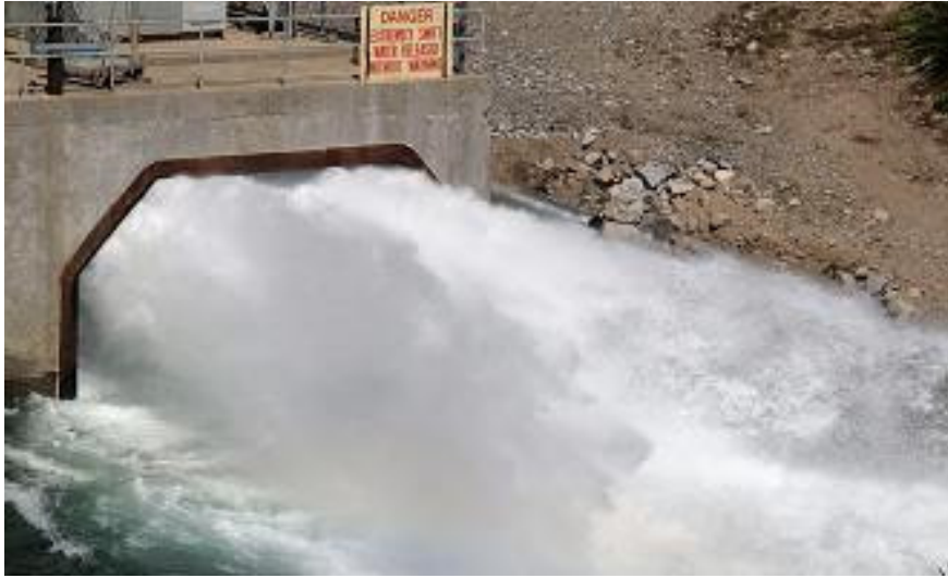
Figure 3.4: An Example of a Tunnel
