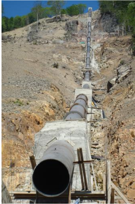
Figure 3.2: An Example of a Penstock
