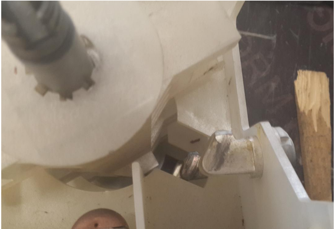
Figure 42: The photo of the earthing contacts
