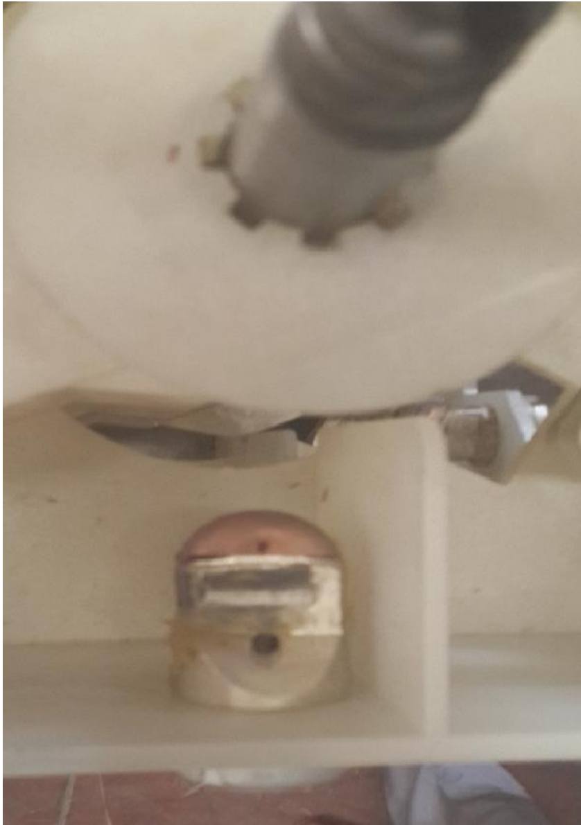
Figure 41: The photo of the busbar contacts and magnet for arc extinguishing
