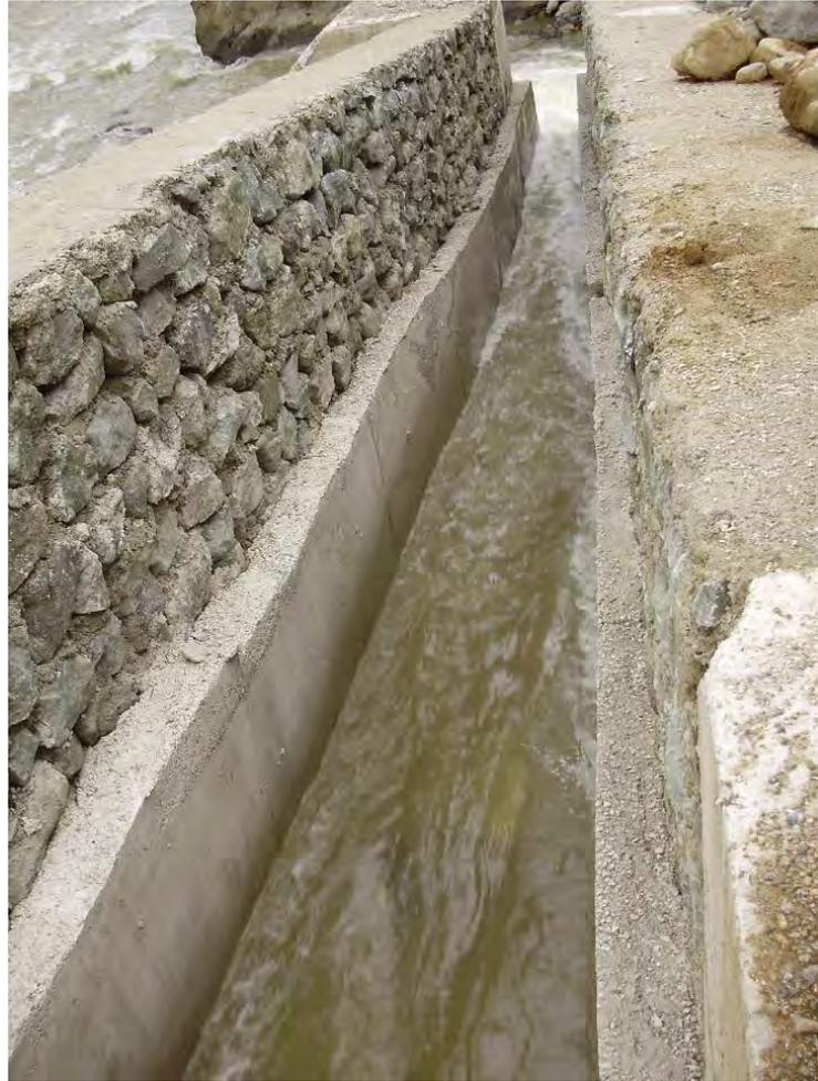
Figure 1.1 An example of inadequate design of fish pass
