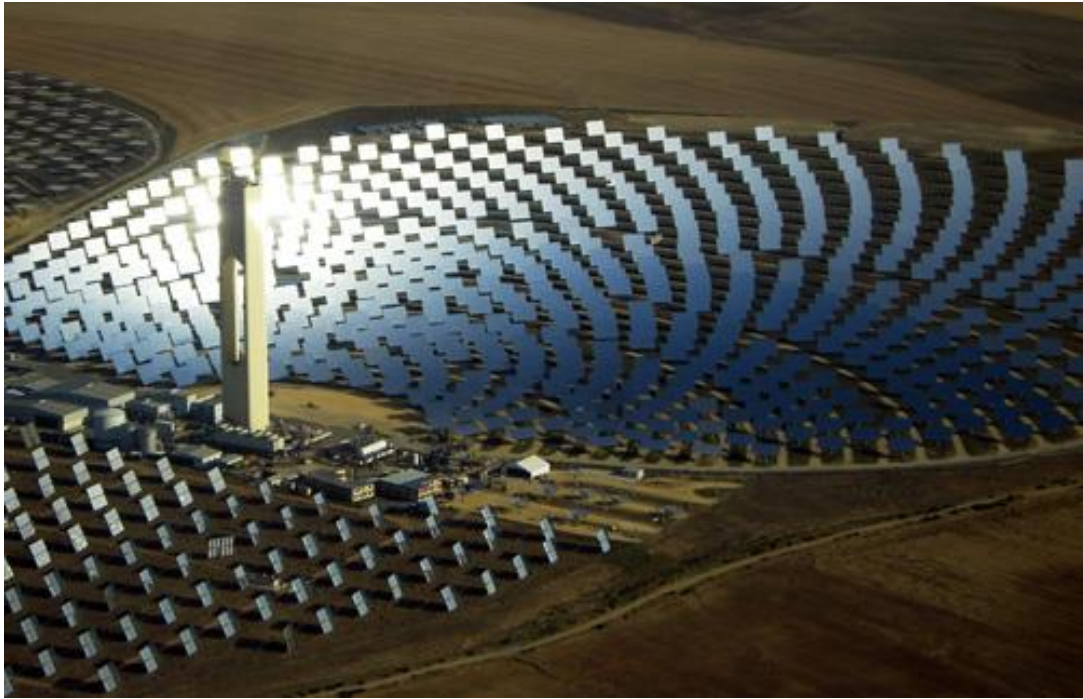
Figure 1.4 Central Receiver Solar Power Plant, (Abengoa, 2012)
