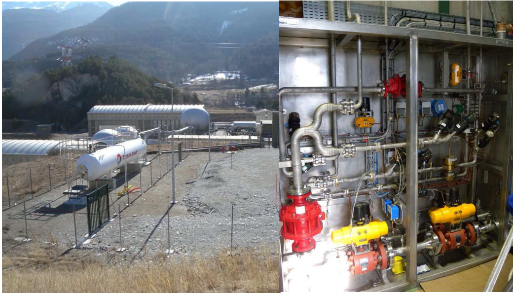
Figure 1.8 Propane Storage and Feeding System [15]
