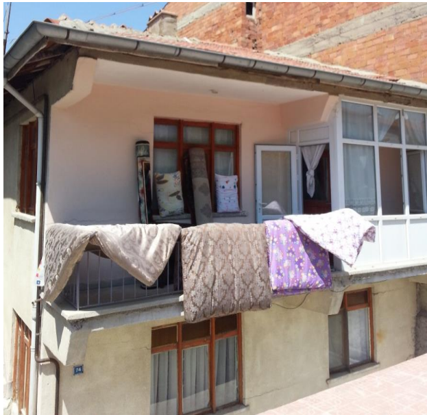
a) Appearance of the building
