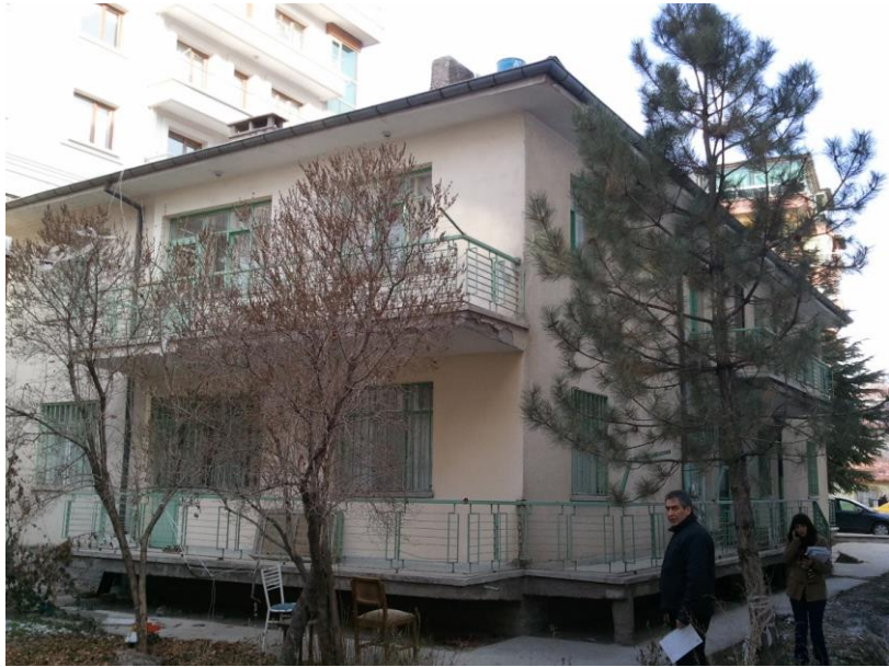
a) Appearance of the building
