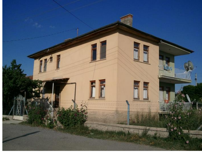
a) Appearance of the building
