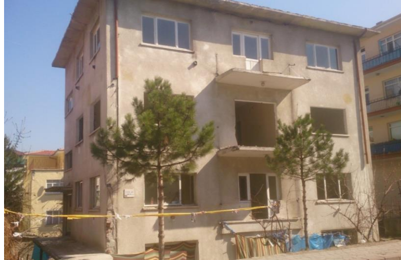
a) Appearance of the building
