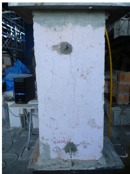
b) Specimen 2* at the end of the test
