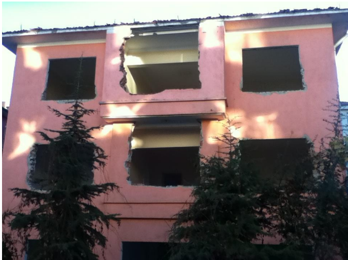
a) Appearance of the building
