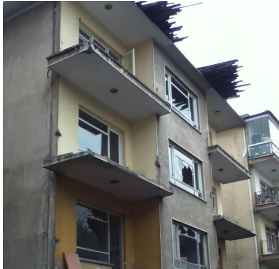
a) Appearance of the building
