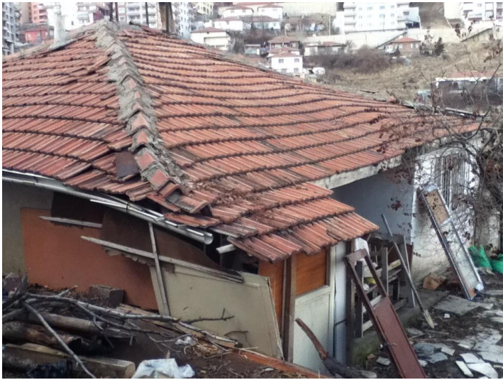
a) Appearance of the building
