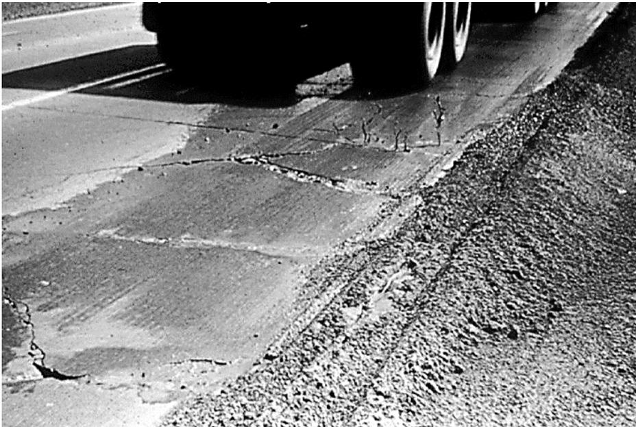
**Figure 2.5** The expulsion of water through the cracks.
