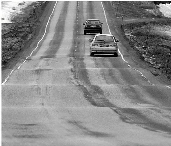
**Figure 2.4** The effect of frost action on asphalt concrete pavements.
