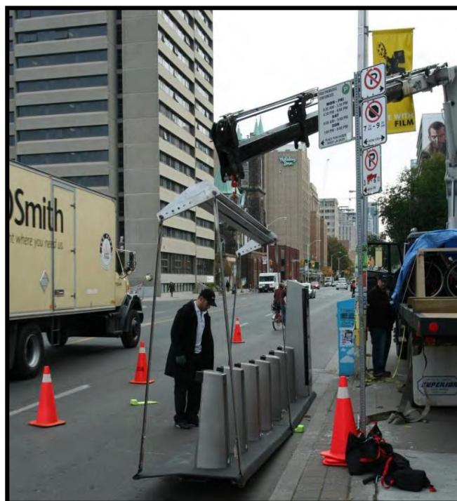
**Figure 15. A Bixi Station Module Being Installed for an Event in Toronto**
