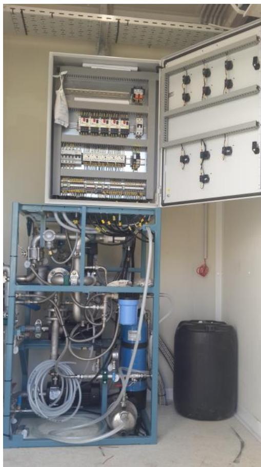
**Figure 5.4:** *De-ionized water cooling system panel*
