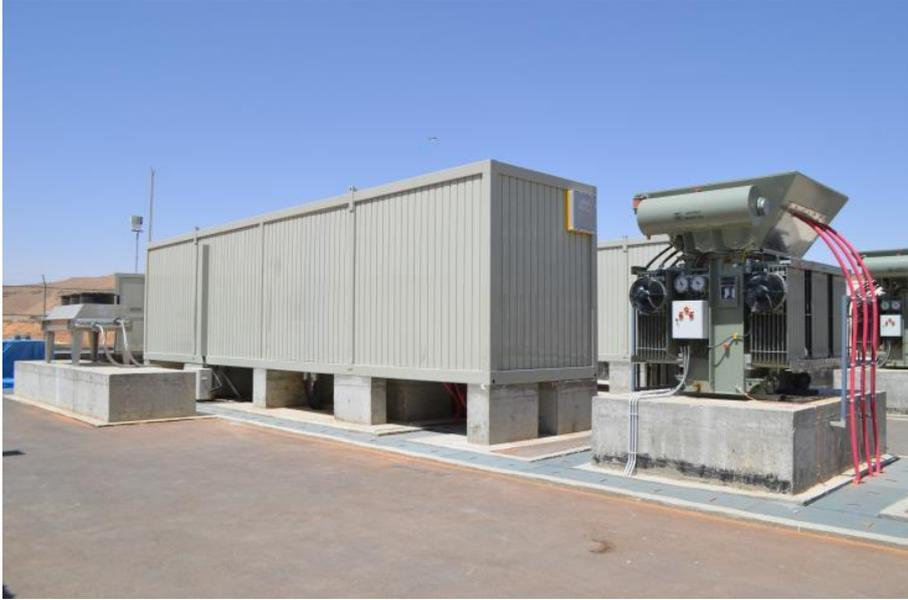
**Figure 5.5:** *SVC container, coupling transformer and heat exchanger*
