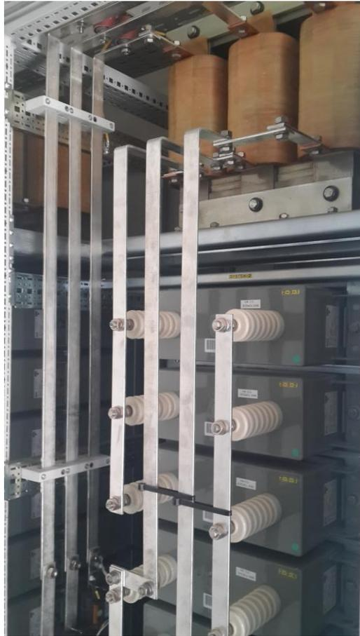
**(b):** *Harmonic filter reactor and capacitor connections*
