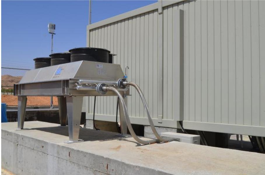
**Figure 5.3:** *De-ionized Water cooling system – heat exchanger*
