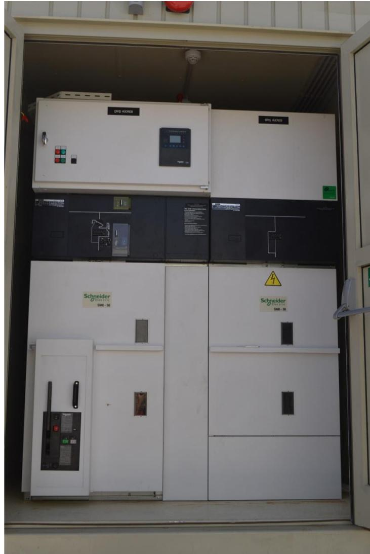
**Figure 3.17:** 36kV circuit breaker cubicle
