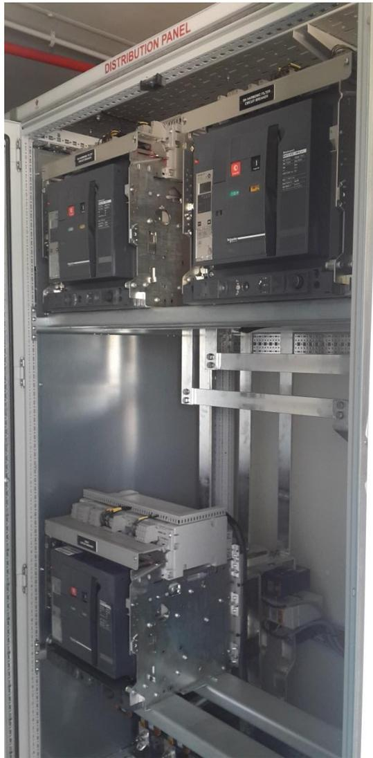
**Figure 3.18:** *1kV circuit breakers mounted on the distribution panel*
