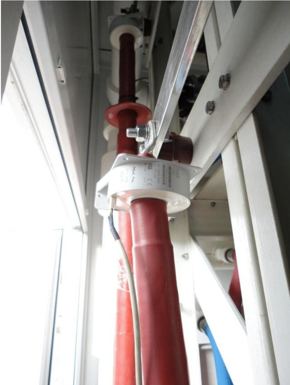
**Figure 4.15 The HECS used in this thesis work for measuring CMC currents**
