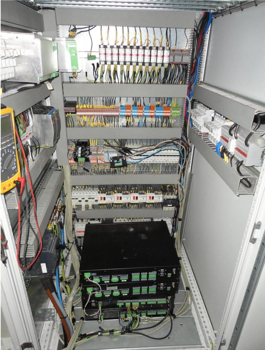
**Figure 4.13 The power quality analyzers used for measurements in scope of the thesis**
