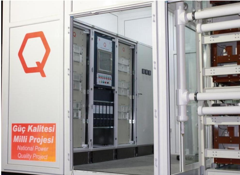
**Figure 2.3 T-STATCOM control cabinets**
