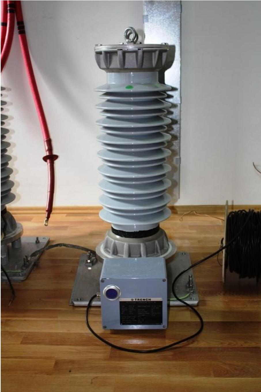
**Figure 4.17 36-kV RCVT column**
