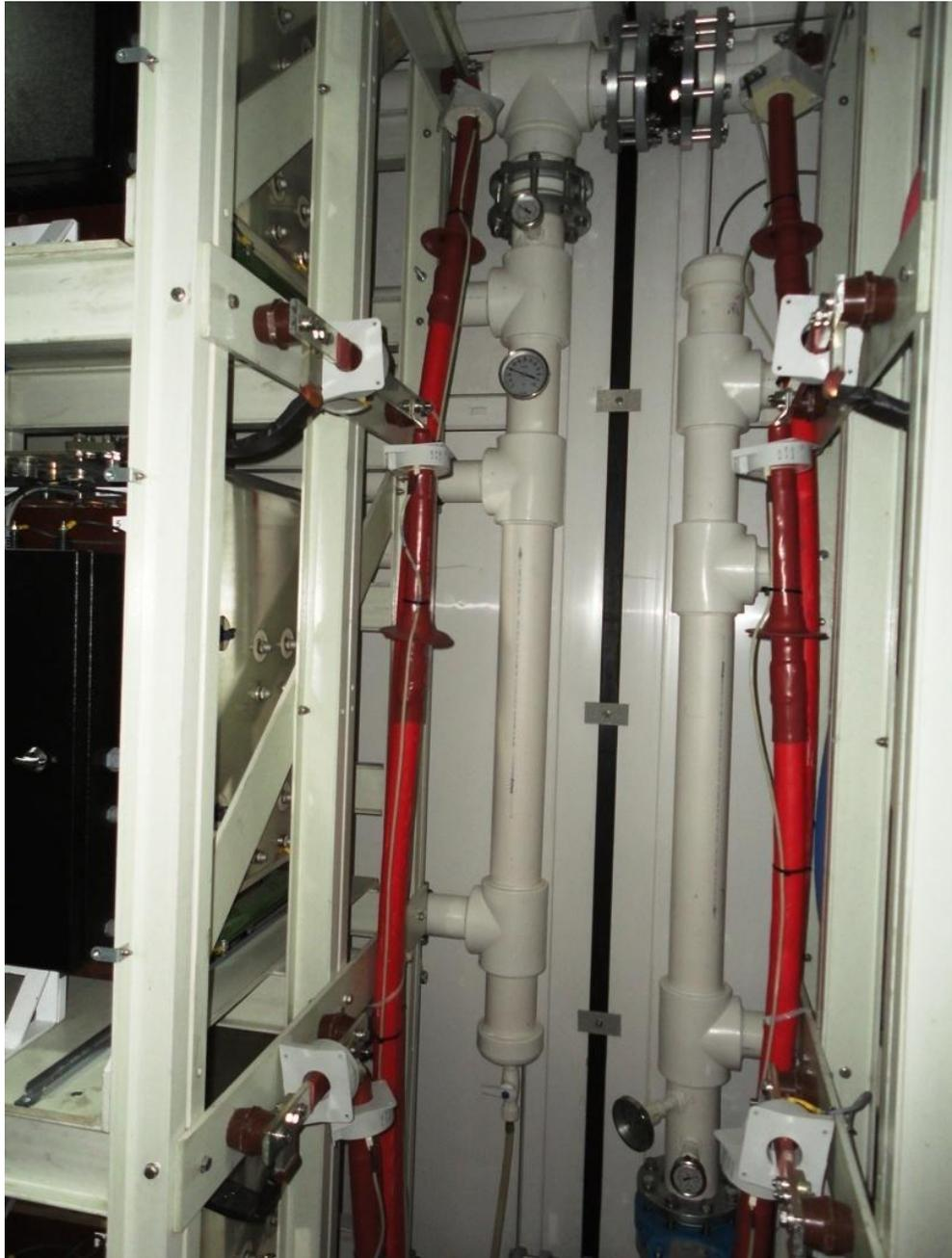
**Figure 4.14 View of HECS sensors on the heads of MV XLPE cables**
