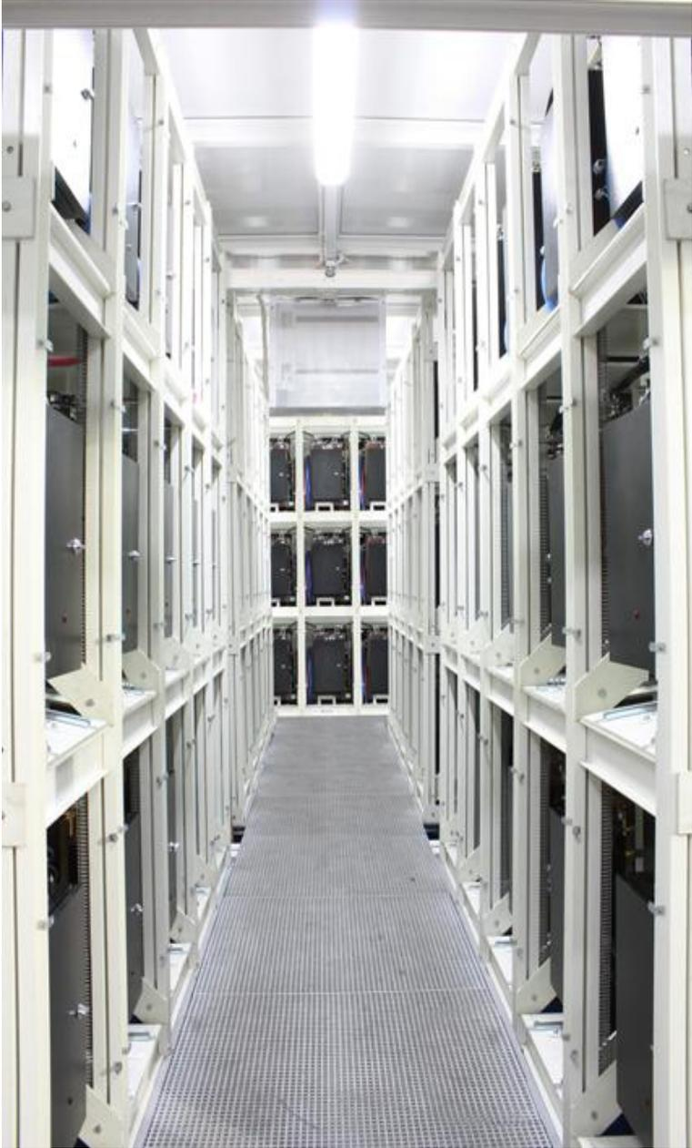
**Figure 2.2 Interior view of T-STATCOM power stage room**
