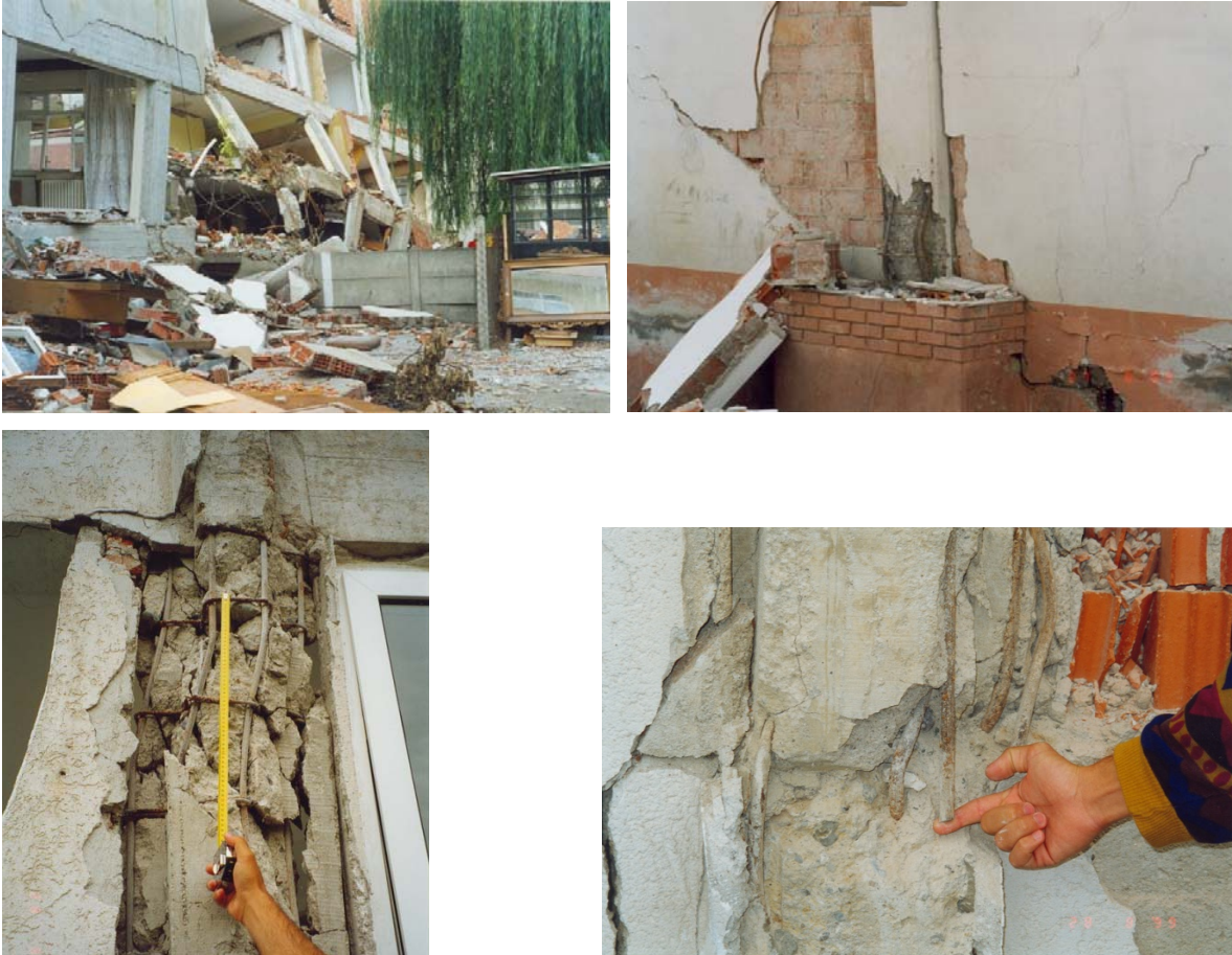
Figure 3.11 Nonductile detailing (photos courtesy of METU-DMC)
