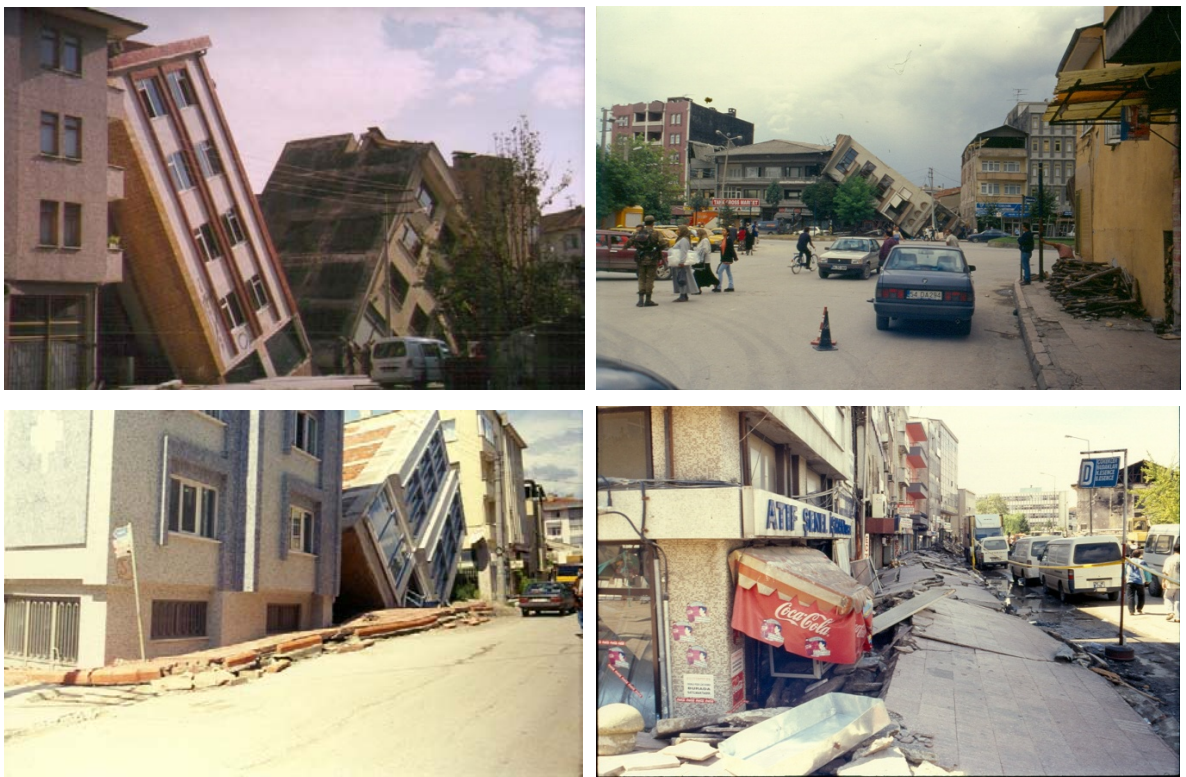
Figure 3.10 Tilting and/or settlement of the buildings (photos courtesy of METU-DMC)
