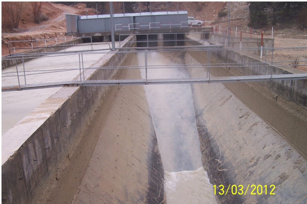
Figure 5.8 Flushing of the right chamber of Birkapılı settling basin
