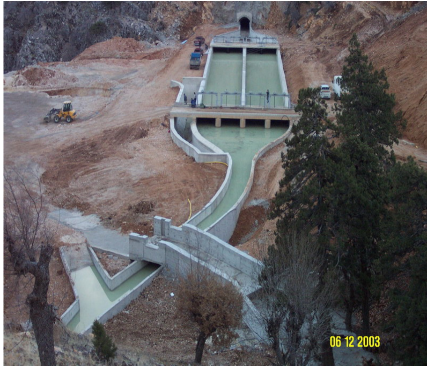
Figure 3.12 Birkapılı settling basin during operation (Mersin, December 2003)
