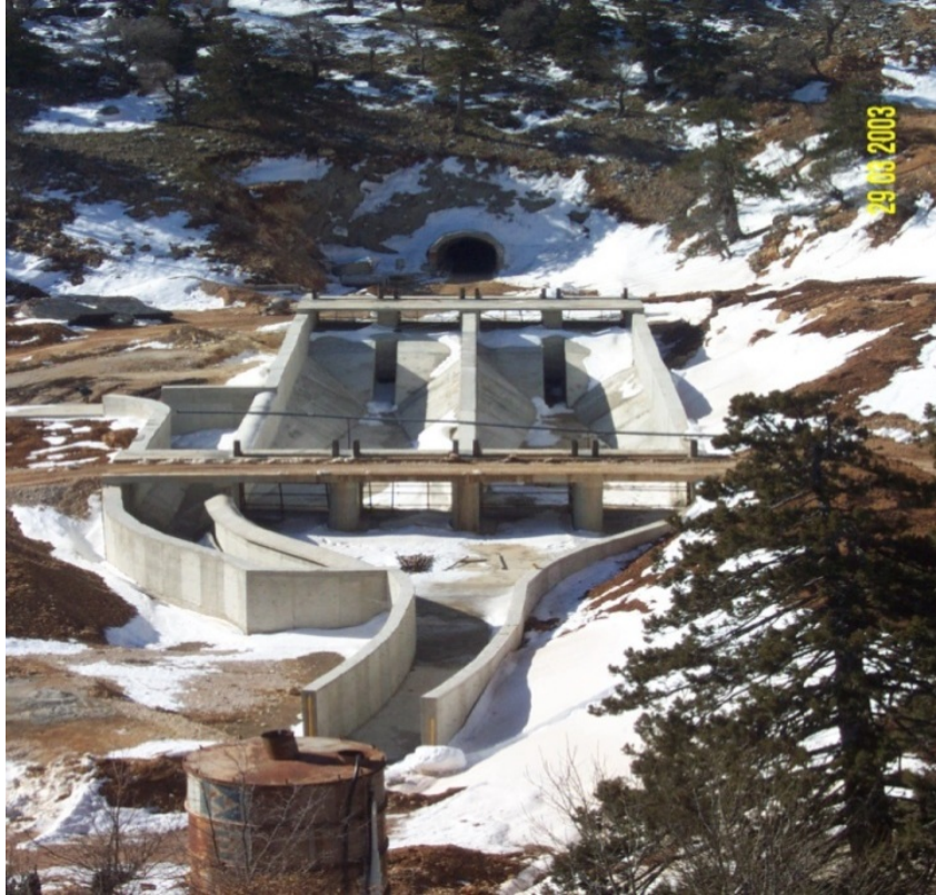
Figure 3.11 Birkapılı settling basin under construction (Mersin, March 2003)
