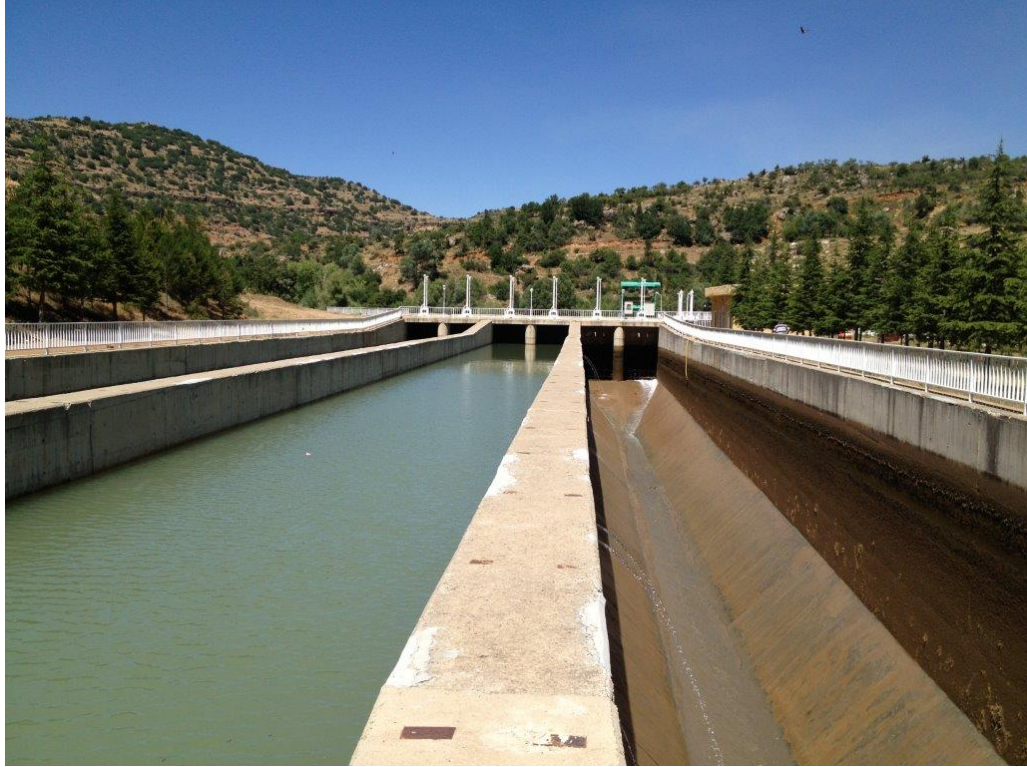
Figure 5.1 Flushing of one chamber of Çamlıca settling basin
