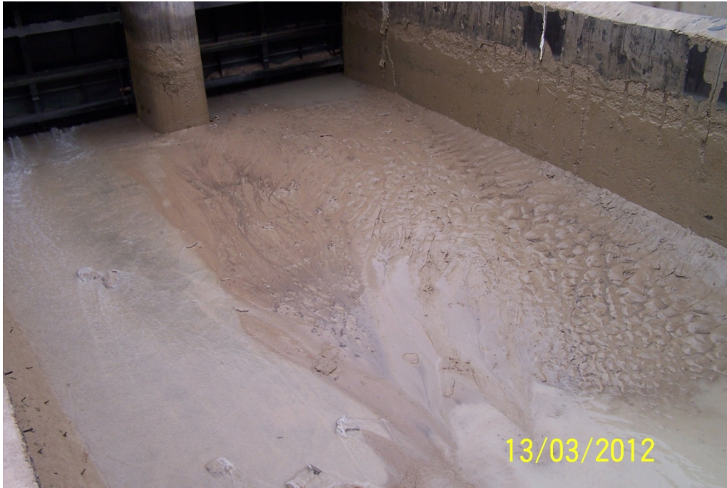
Figure 5.9 The entrance of Birkapılı settling basin after flushing
