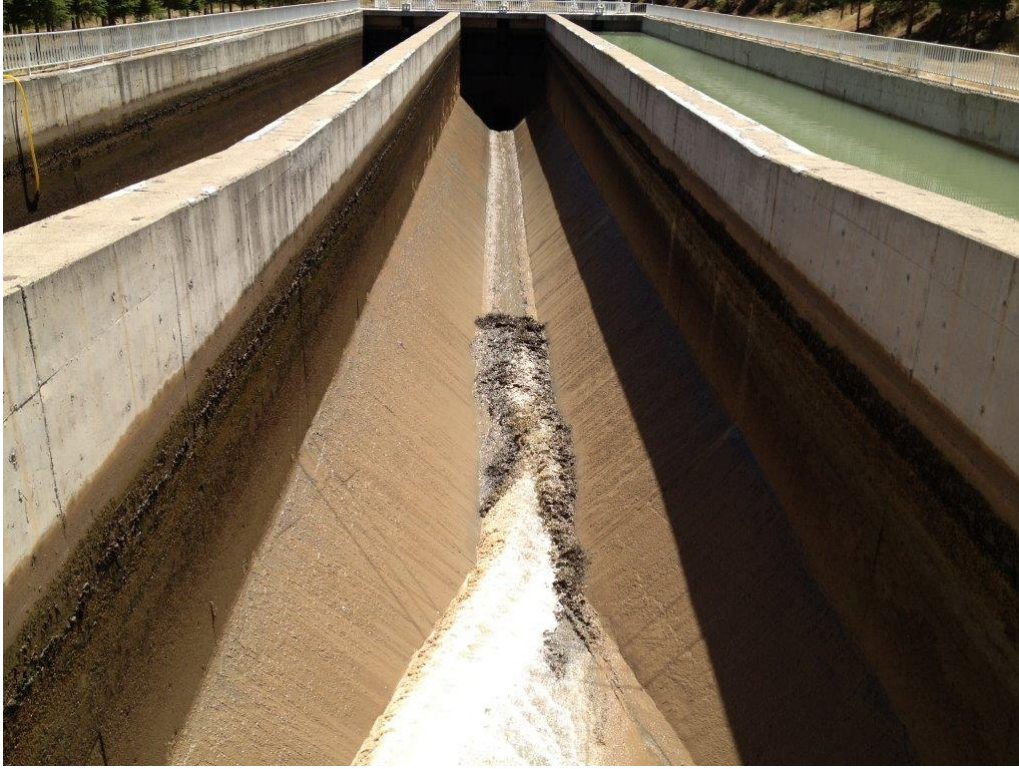
Figure 5.3 Çamlıca settling basin during flushing
