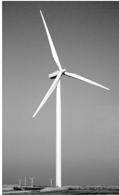
Figure 1.3: Multi Mega Watt HAWT (Rotor Diameter: 107m and Rated Power 3.6MW) [3]
