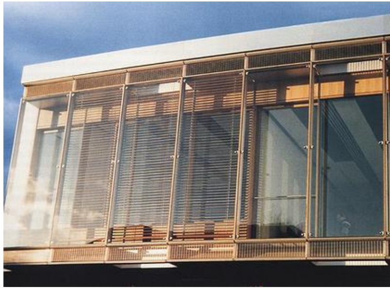
Figure 2.3 The box type window (Source: Berezovska, 2011)
