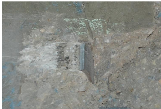
Figure 1.17 Channel Fracture – Concrete Slab
