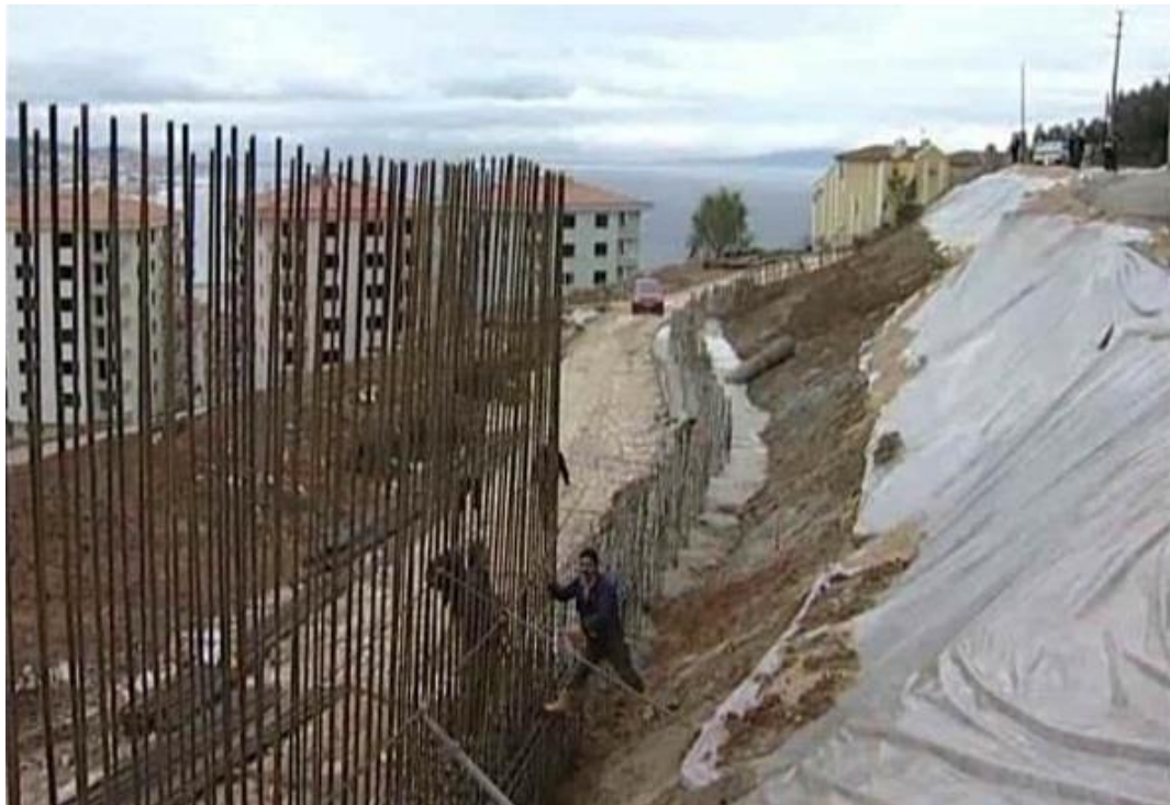
Figure 2.1 a) Landslide stabilization with reinforced concrete piles in Güzelyalı, Bursa
