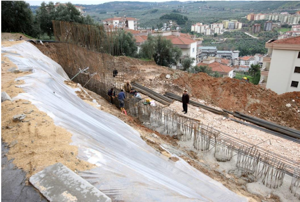
Figure 2.2 b) Landslide stabilization with reinforced concrete piles in Güzelyalı, Bursa
