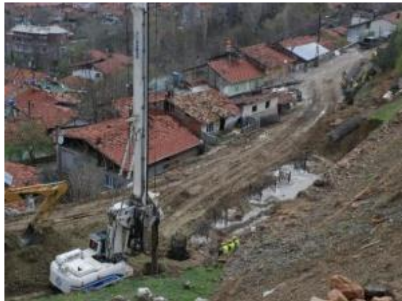
Figure 1.1 Landslide stabilization with passive piles for a freeway in Tokat
