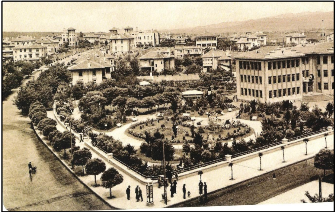
Figure 4.29 Kızılay Bahçesi in 1935. Source: MEB, 2007.
