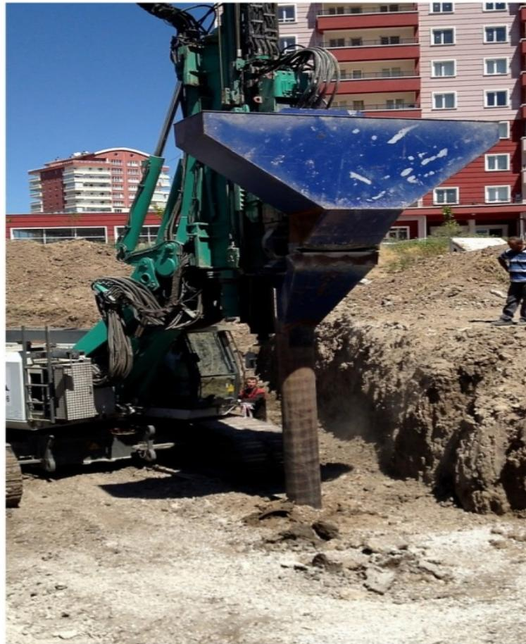
Figure 3.2 Construction of the rammed stone columns at field
