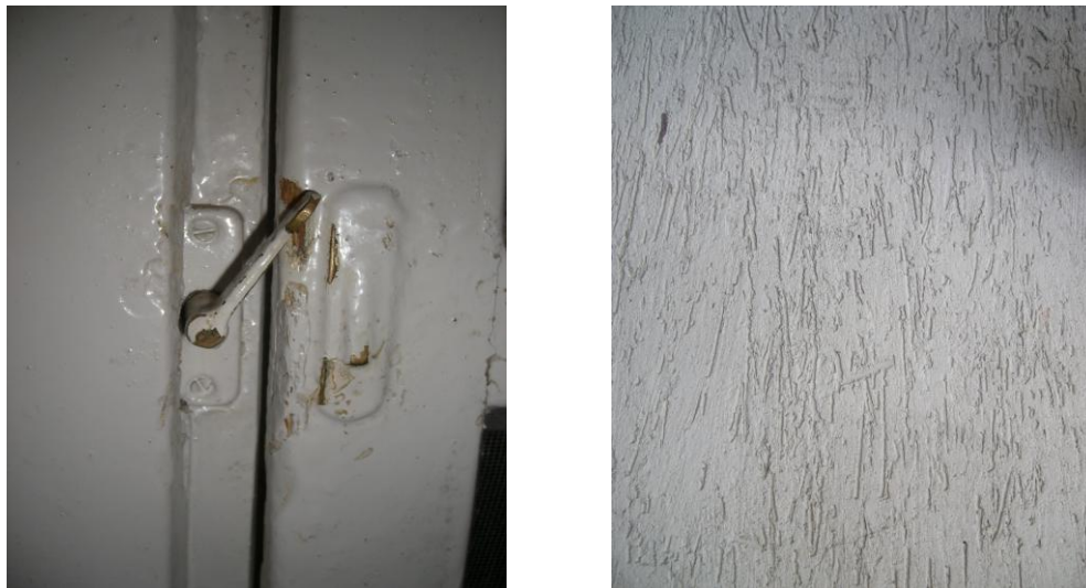
Figure 102. The original locking detail in the double storey dwellings of officers (left) and the texture of the artificial stone plaster, seen on the exterior walls (right) (Source: Author)
