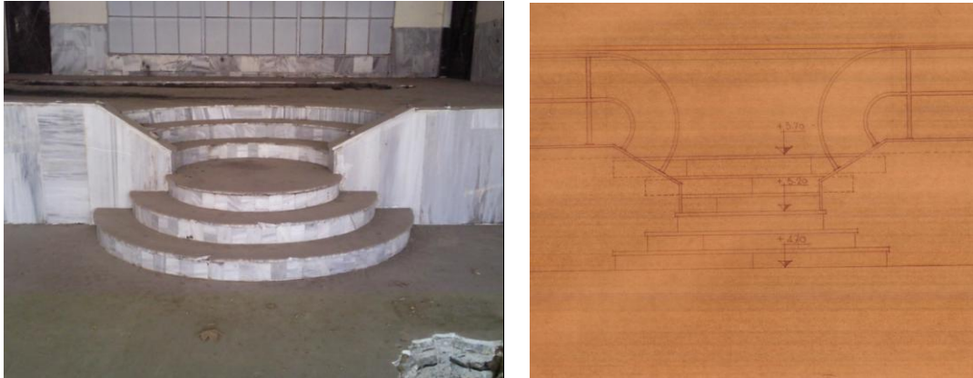
Figure 84. Photograph of the circular formed stair in the boiling and fermentation building (left) and the original detail drawing of Ernst Egli in 1937 (right). (Sources: Author and TTA Archive)
