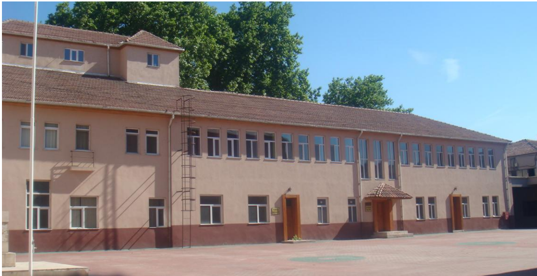
Figure 37. Exterior photograph showing the north facade of the old factory building (Source: Author, 2012)
