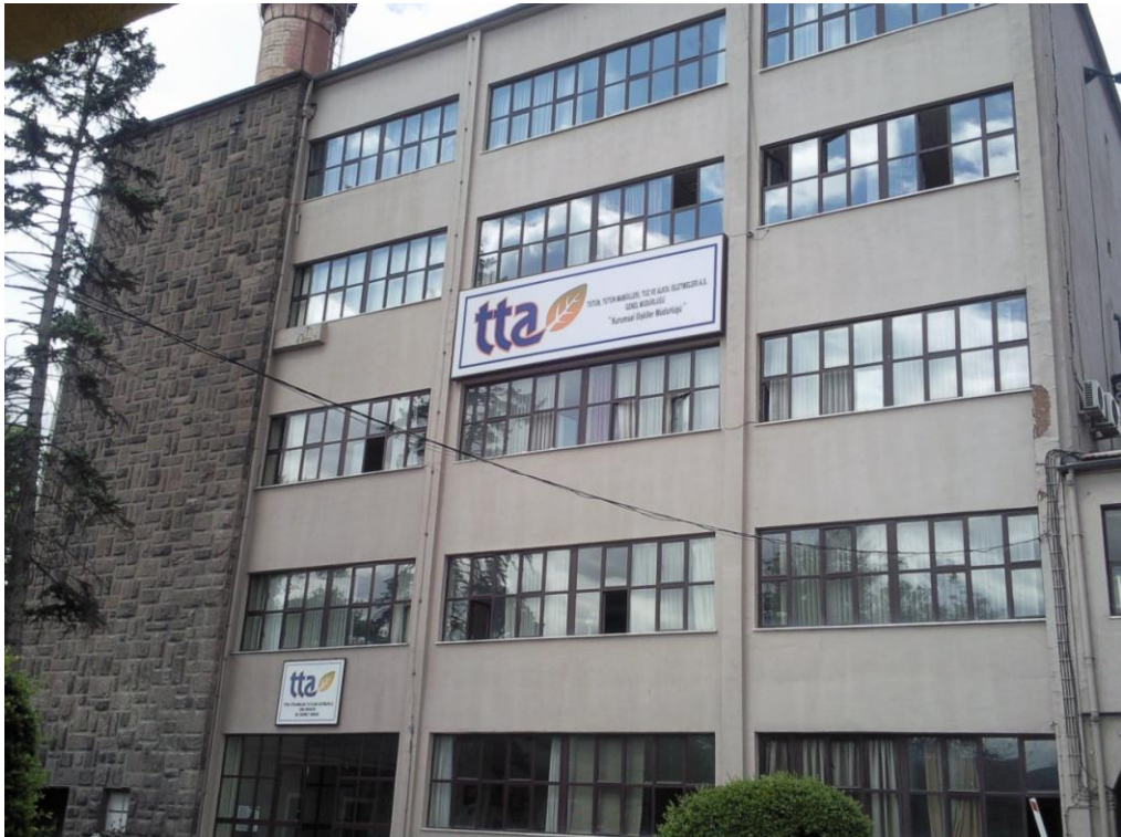
Figure 59. Exterior photograph of the malt building (Source: Author, 2012)
