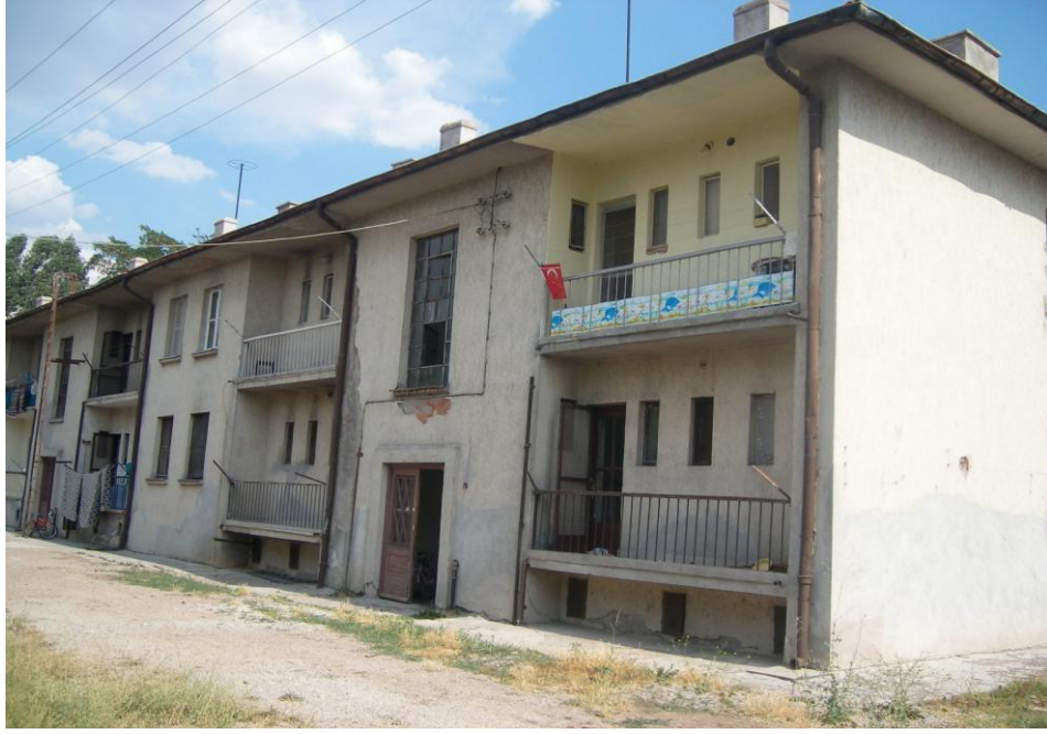
Figure 98. The exterior photograph from the north facade of the double storey dwellings of officers (Source: Author)
