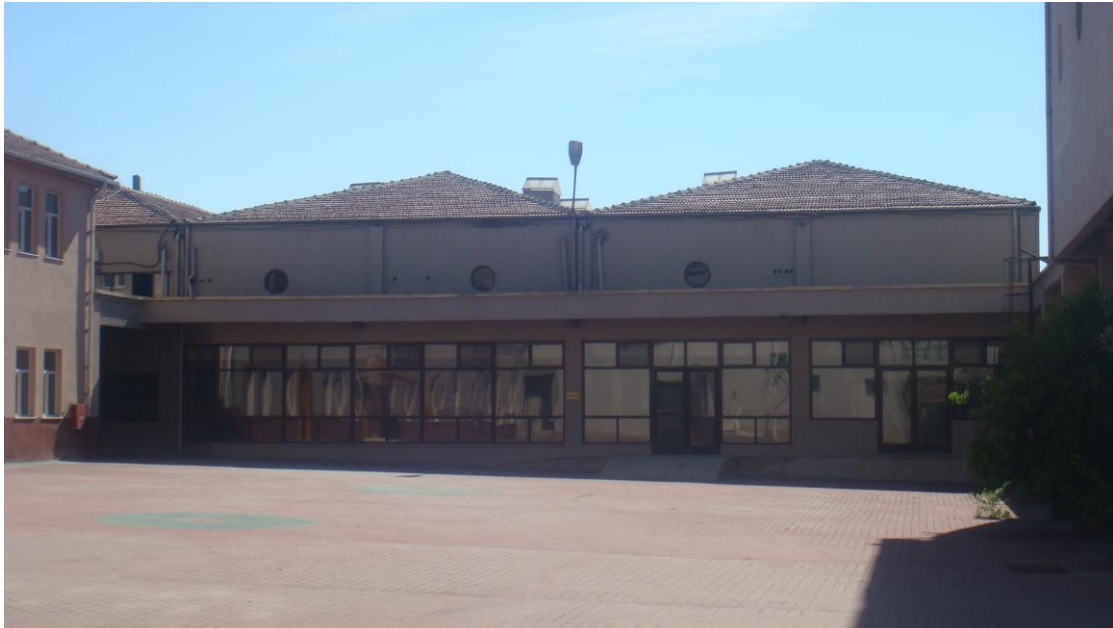
Figure 66. Exterior photograph of the beer filling building (Source: Author, 2012)
