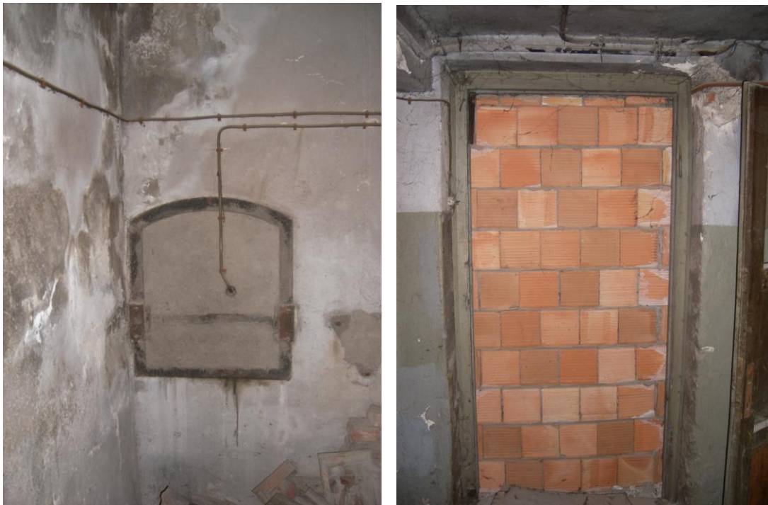
Figure 46. The closed openings in the production part of the old factory buildings (Source: Author, 2012)
