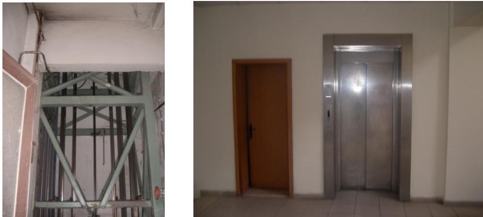
Figure 64. The toilets and elevator, which were added in 2001, were constructed with steel frame system (Source: Author, 2012)
