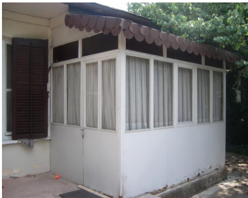
Figure 109. The additional timber construction which is not seen on the original drawings (left), the altered and enlarged window with altered iron balusters added in recent times (right) (Source: Author)
