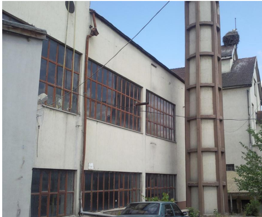
Figure 75. The exterior photograph of the boiler house and chimney (Source: Author)
