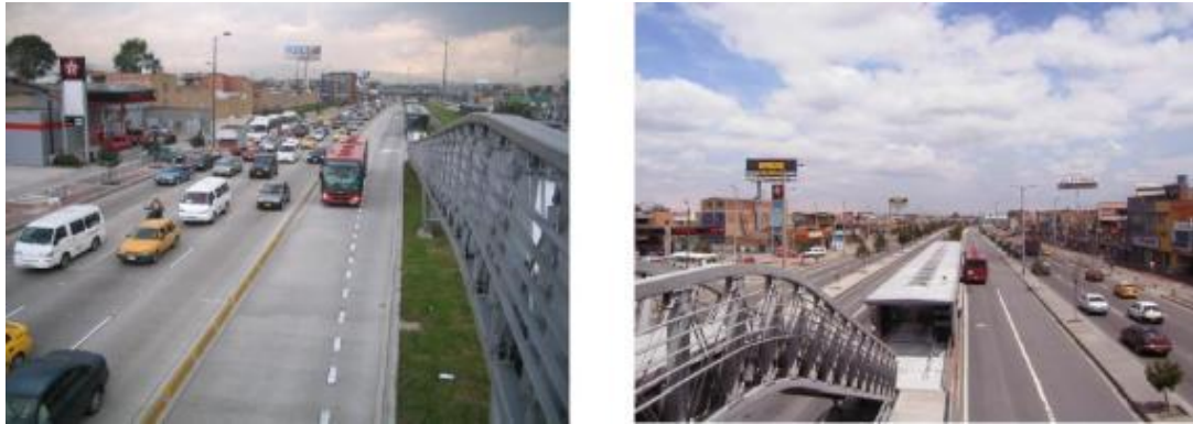
Figure 26: Running ways and overpass examples in TransMilenio
