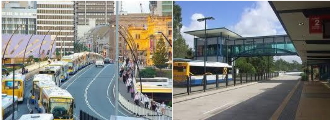
Figure 20: Brisbane BRT running ways and interchange stations
