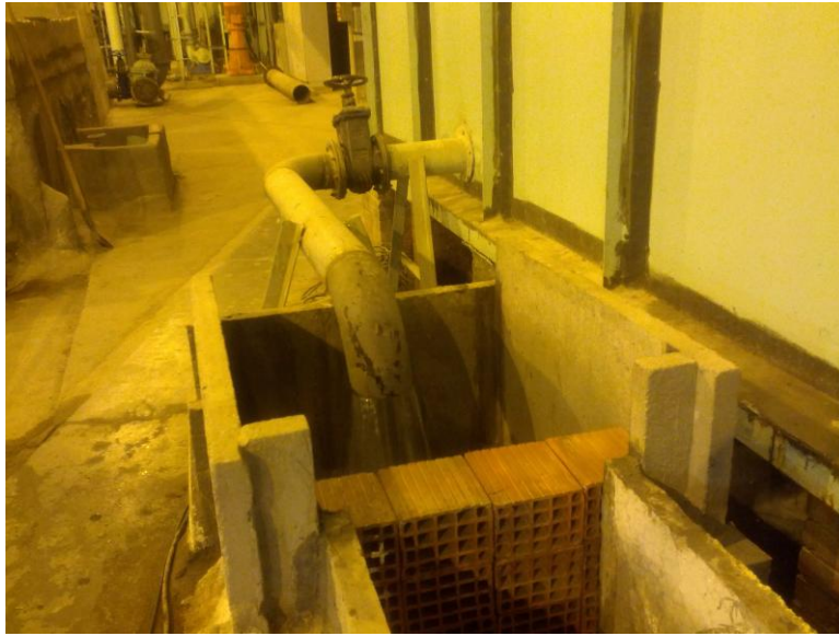
Figure C.9: Outflow pipe and settling pool
