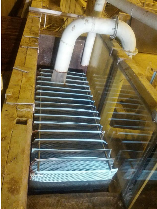
Figure C.5: Inflow pipe and steel meshes
