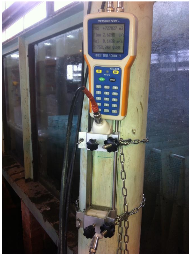
Figure C.11: The flowmeter that is installed on inflow pipe
