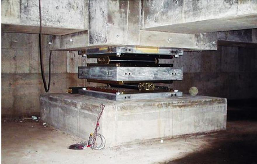
Fig. 2.2 Seismic isolation by mechanical devices
