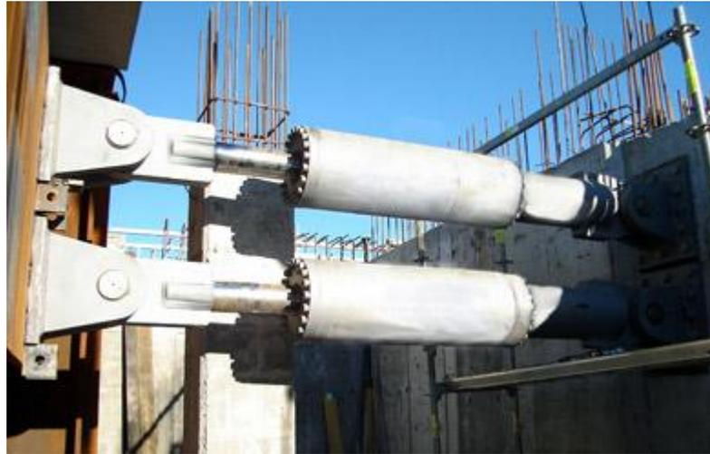
Fig. 2.3 A structure isolated by hydraulic dampers
