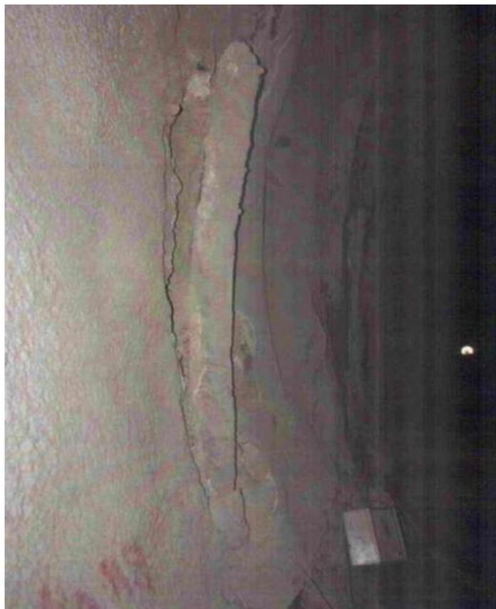
Figure 3.5 Deformations in shotcrete lining and steel supports at bench level (source: SIAL Report, 2010)
